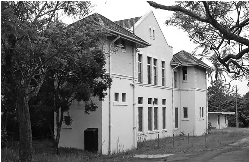
Figure 3: Noble House, Wolston Park Hospital Complex, 2004.
