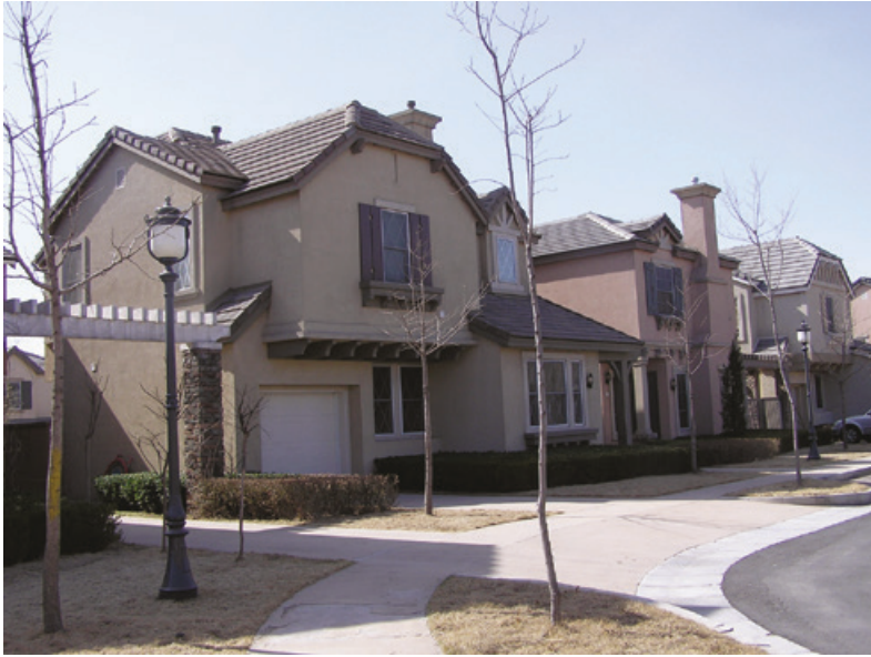
Figure 4.5 A rather exotic style as seen in China, but quite ‘ordinary’ detached houses in North America, in the ‘Orange County’ estate, Beijing. Taken in 2004.
