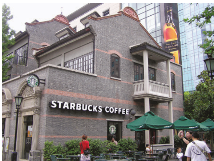
Figure 2.12 The redevelopment of alleyway housing into an entertainment and shopping district in Xintiandi, Shanghai. The photo shows the reconstruction of ‘stone portal gate’ housing into a cafeteria, bars, restaurants and boutique shops. Taken in 2003.
