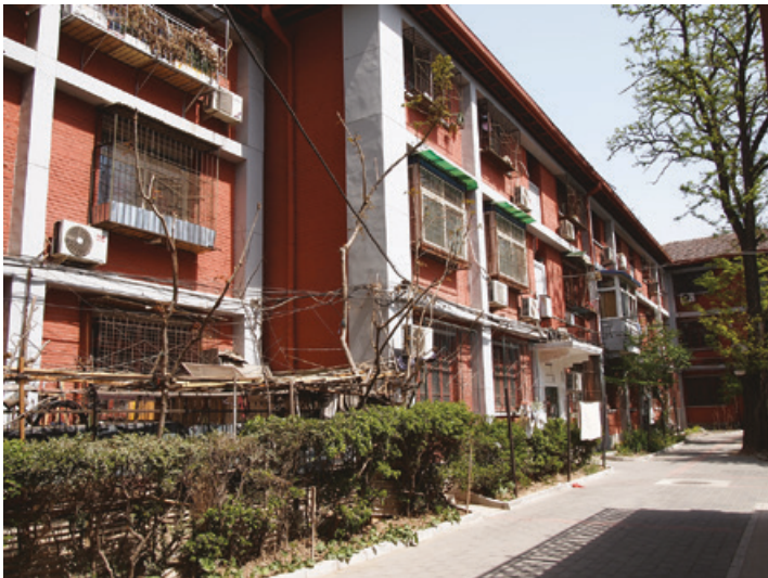
Figure 1.5 The work-unit compound of Baiwanzhuang, Beijing, before the area was demolished in 2014. The quality of housing was relatively higher as it was for the staff living quarters of the central government ministries. The layout was influenced by the Soviet super neighbourhood block. Taken in 2014.
