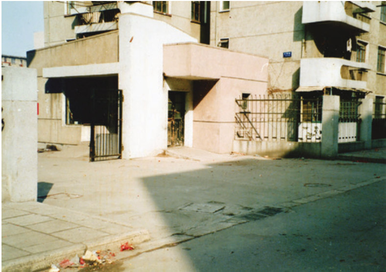
Figure 2.9 The southern gate of the inner compound reserved for work-unit staff in the Fifth Village, Nanjing. Although the gate is not strictly controlled, it is served with a security guard room. This rather rudimentary ‘gated community’ reveals the attempt to maintain social order through management rather than neighbourhood self-governance in an urbanising mobile society in China. Taken in 1997.
