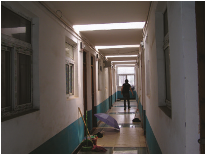
Figure 3.8 The decent living conditions of purpose-built apartments constructed by small developers in Tangjialing, Beijing. The photo shows how natural light is introduced into the corridors. Taken in 2010.
