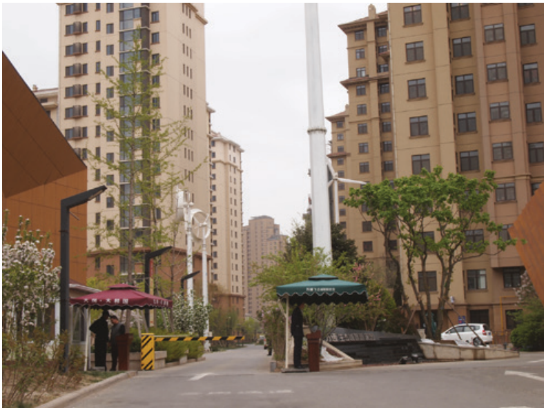
Figure 1.8 An ordinary commodity housing estate in Tianjin Sino-Singapore Eco-city. The area was previously low land in an industrial area. The photo shows some modest security and the gate. Taken in 2014.
