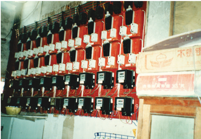
Figure 2.2 Subdivision of single-family lane houses into multiple occupancies, making the courtyard extremely crowded. The photo shows many electric meters for this lane house near Tianjin Road, Shanghai. Taken in the late 1990s.
