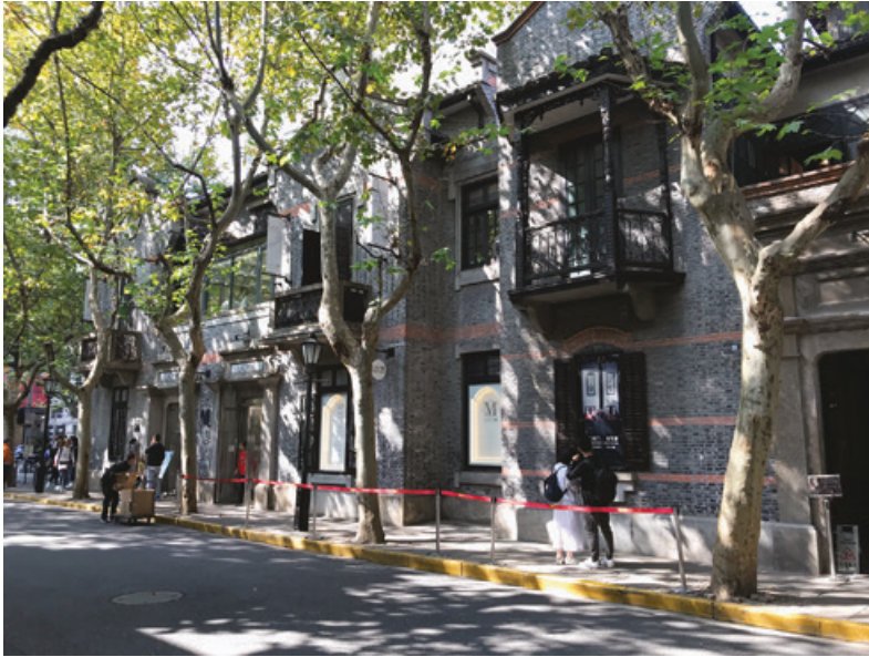
Figure 2.13 The traditional shikumen style housing in the Xintiandi area, Shanghai. The shikumen housing has been carefully refurbished since the late 1990s. The photo shows the ‘stone portal gates’ leading to an internal courtyard. The style is actually a hybrid of the traditional Chinese courtyard and Western terraced housing in order to be land efficient with increased density. Taken in 2019.
