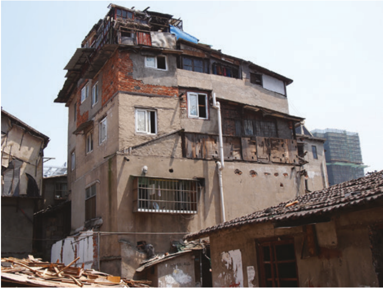
Figure 3.13 After many informal houses were demolished, some original self-extension became visible. The building was dangerously increased to four and a half floors. The original ground floor house was still visible and had a rather weak foundation and structure. Taken in 2013.
