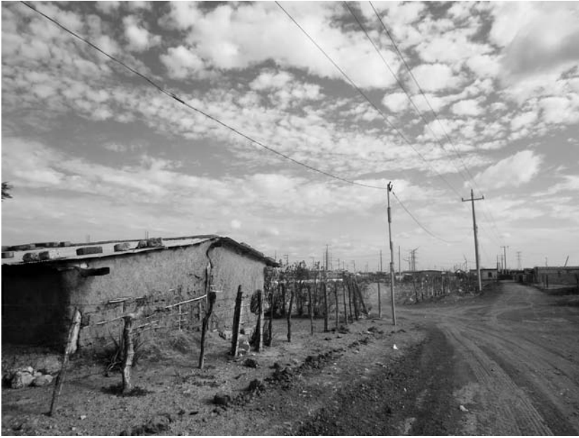
FIGURE 2.1. House, road, electric infrastructure, and turbines, La Ventosa
