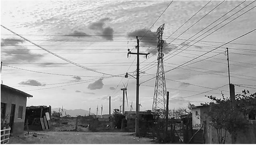
FIGURE 1.5. Turbines and high-tension wires, La Ventosa
