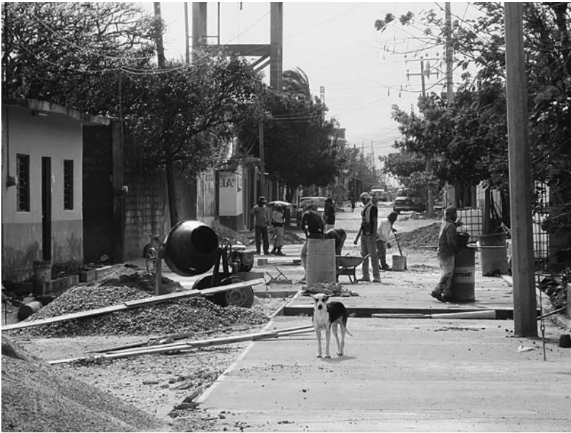
FIGURE 3.3. Paving the streets of La Ventosa
