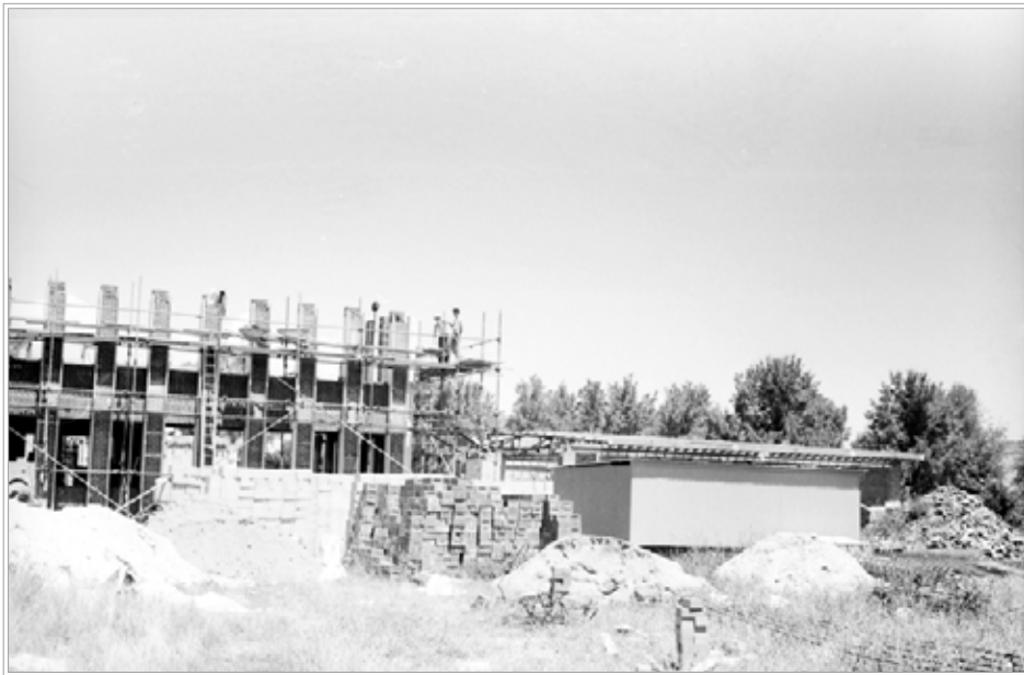
Plate 3.5 The new wing of the Old Geology Building under construction
