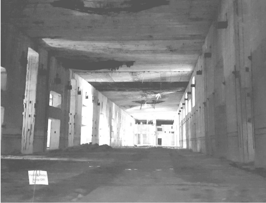
Figure 6.7: Ruined part as seen from visitor's area.
