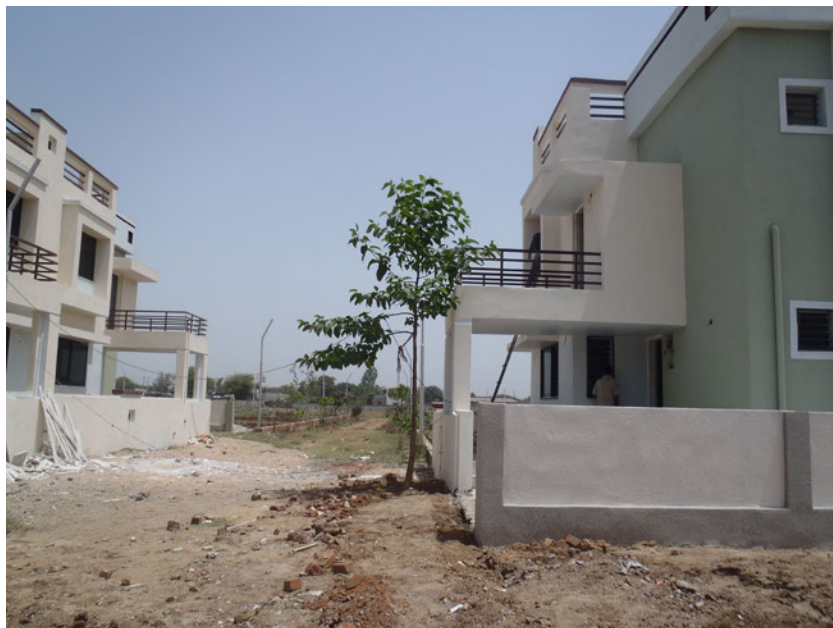
FIGURE 2.1. Sprawling outskirts of Anand, with newly constructed houses, plots waiting for development, and mostly unpaved roads. (Photo by the author, 2012.)
