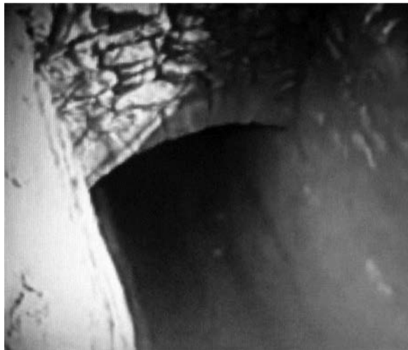
Figure 18.17 The shaft in the underground aqueduct constructed under Morosini's orders (with permission of E.G. Chalkiadakis)
