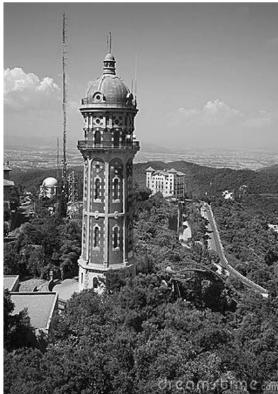
Figure 19.9 Tibidabo water tower (commissioned in 1905) in Collserola range (Source: Water tower Tibidabo Barcelona Spain, Stock Photo)
