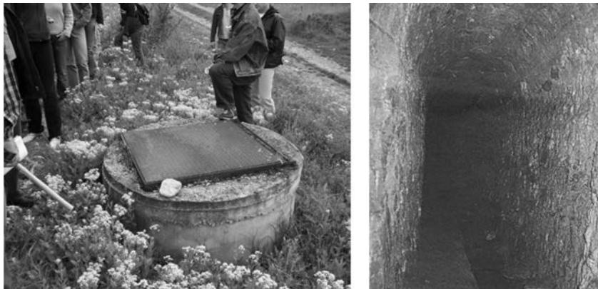
Figure 4.10 Left: The initial well (shaft) of a qanat in Nea Zichni (with permission of K. Voudouris). Right: The tunnel of a qanat at Chortiati, Thessaloniki constructed in the 18th century (with permission of K. Voudouris)
