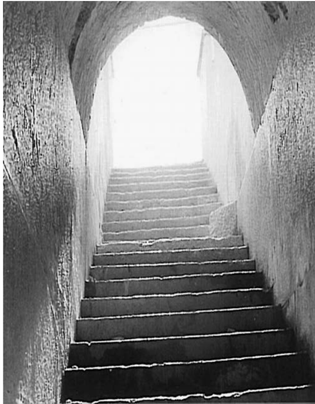
Figure 5.16 Access way to the sewerage networks
