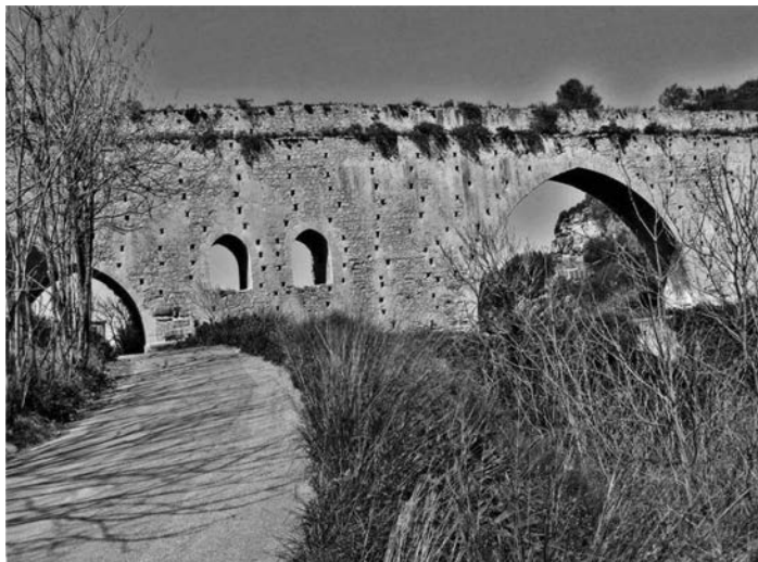
Figure 18.19 Bridge – aqueduct at Hagia Irini, Spilia (with permission of E.G. Chalkiadakis)
