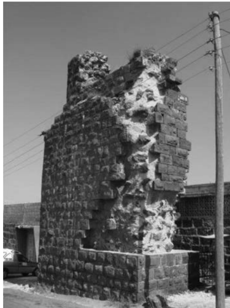
Figure 13.4 Remains of an aqueduct bridge within the city of Shahba
