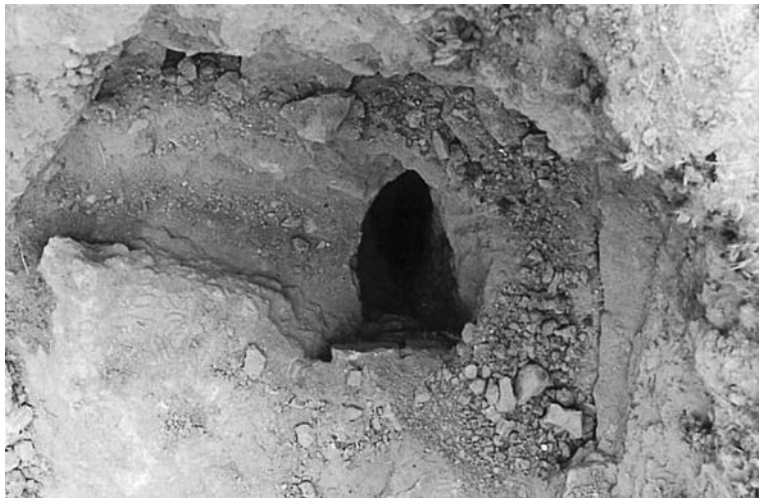
Figure 5.18 Lower segments of the conduits at the sewage outlet
