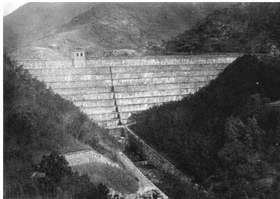
Figure 8.47 Dam (1883–1888) of the Tai Tam Upper Reservoir in Hong Kong (photo of 1907) (Ho Pui Yin, 2001)
