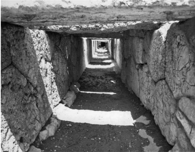
Figure 16.23 Interior view of the Great Drain: ASCSA, image 1997.04.0290
