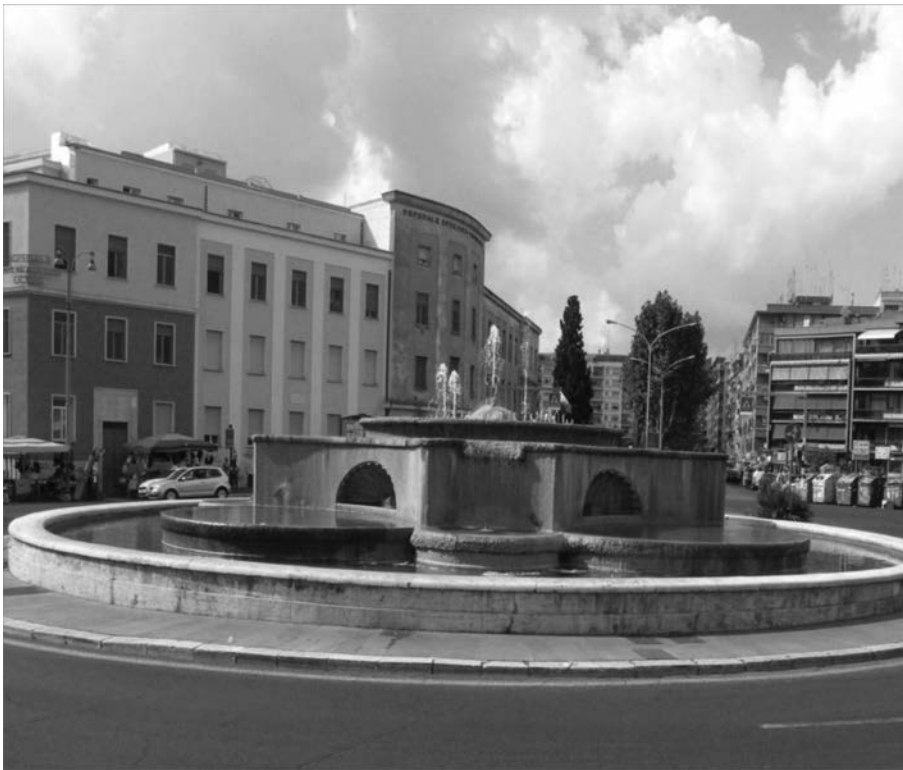
Figure 17.21 Fountain in Piazzale degli Eroi as “display” of the Peschiera Aqueduct ( photo by R. Drusiani )
