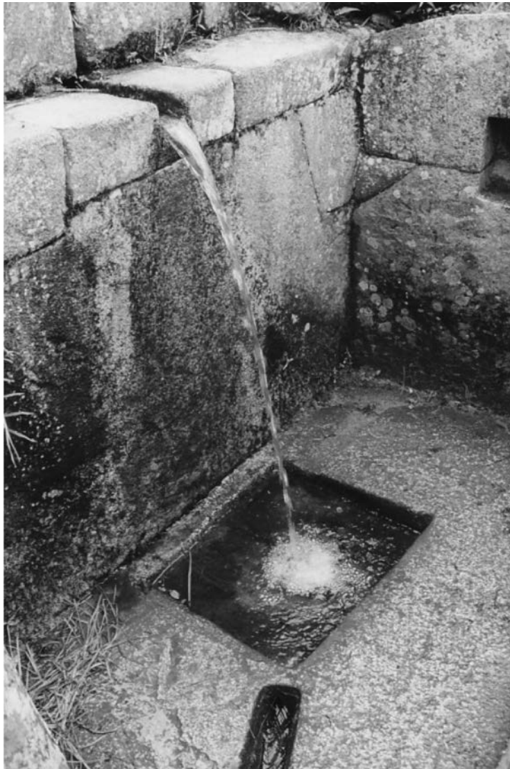
Figure 11.18 Machu Picchu, Peru. Detailed view of the so called “ceremonial centre”, where rituals and cults dedicated to water could have taken place (Photograph taken by the author in October 2000). Note the walls of perfectly matching stones, build without the use of any mortar, and also the jet of water gently falling into a carved basin and continuing its course through a small channel carved on the same stone
