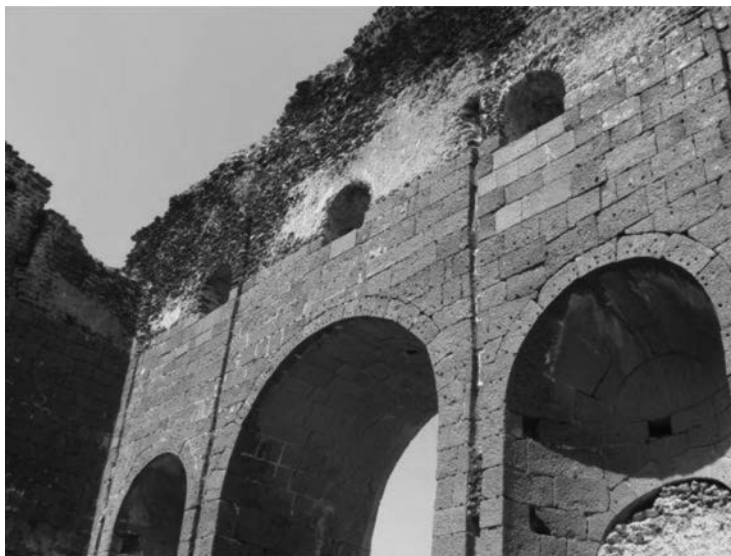
Figure 13.33 Philippopolis baths. Notches can be observed on the room walls
