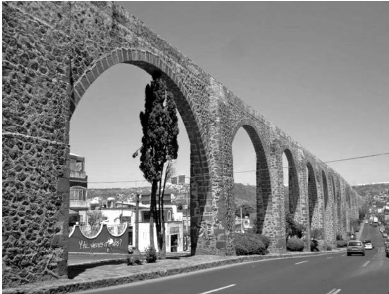
Figure 15.14 Queretaro Aqueduct, Mexico. The aqueduct was constructed between 1726 and 1735, bringing water from the springs of La Canada to the Convent of La Cruz protecting the valley of Carretas. The structure consists of 74 arches with a radius of 5.85 m and a maximum height of 28.5 m (with permission of Karla S. Estrada Herzfeld)
