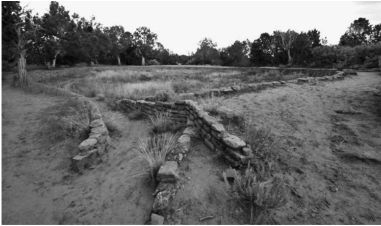
Figure 15.6 Far View Reservoir at Mesa Verde National Park. In the foreground is the restored intake structure (canal) into the reservoir (with permission of L.W. Mays)
