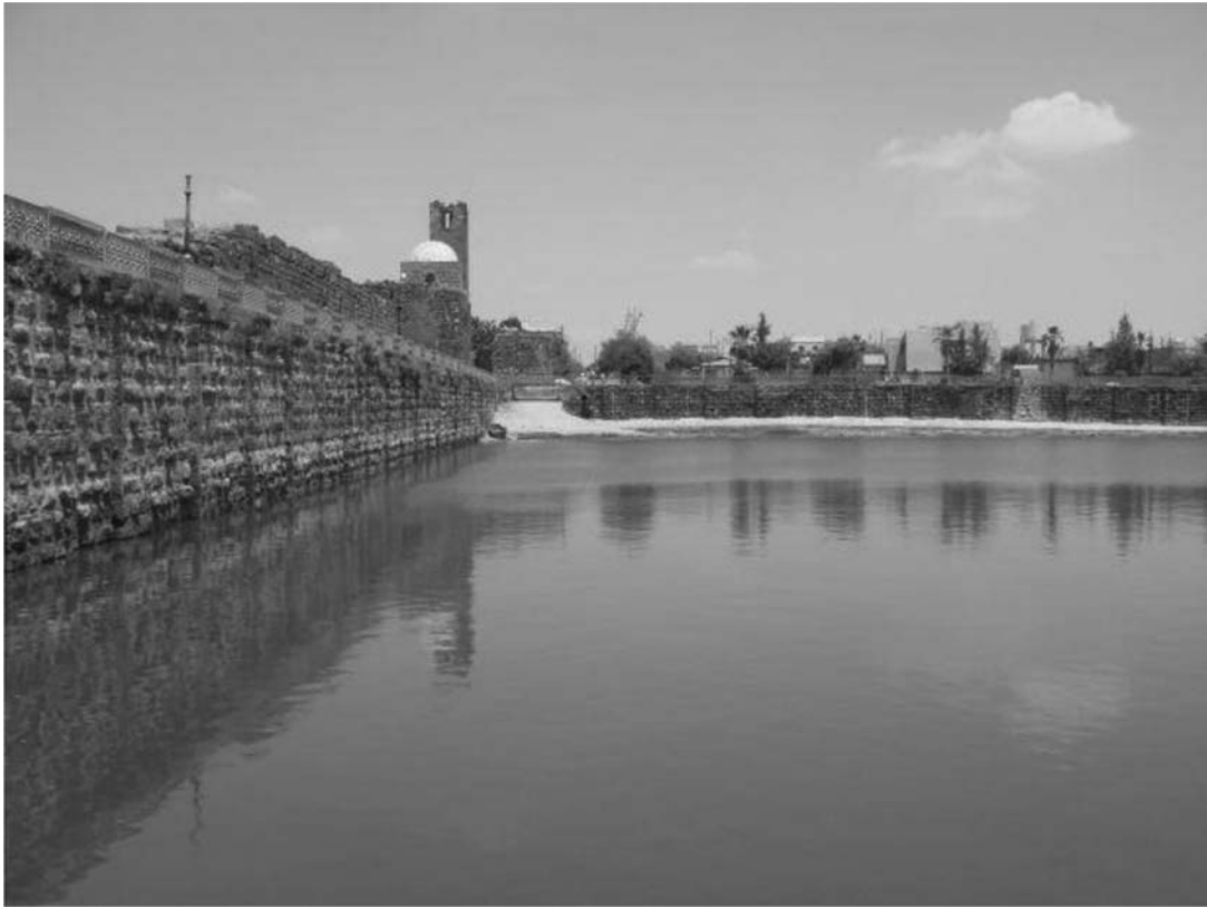
Figure 13.38 Large cistern in the north-east area of Bosra
