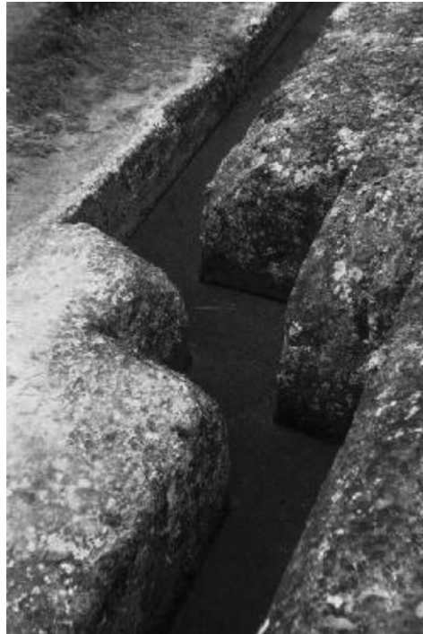
Figure 11.7 Detailed view of the first section of the Cumbe Mayo aqueduct carved on volcanic rock
