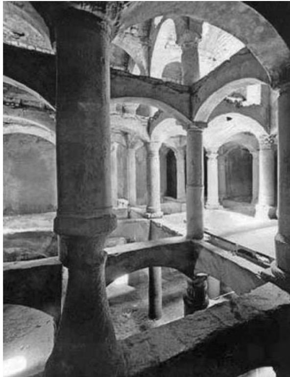
Figure 6.10 Inside El-Nabih Cistern
