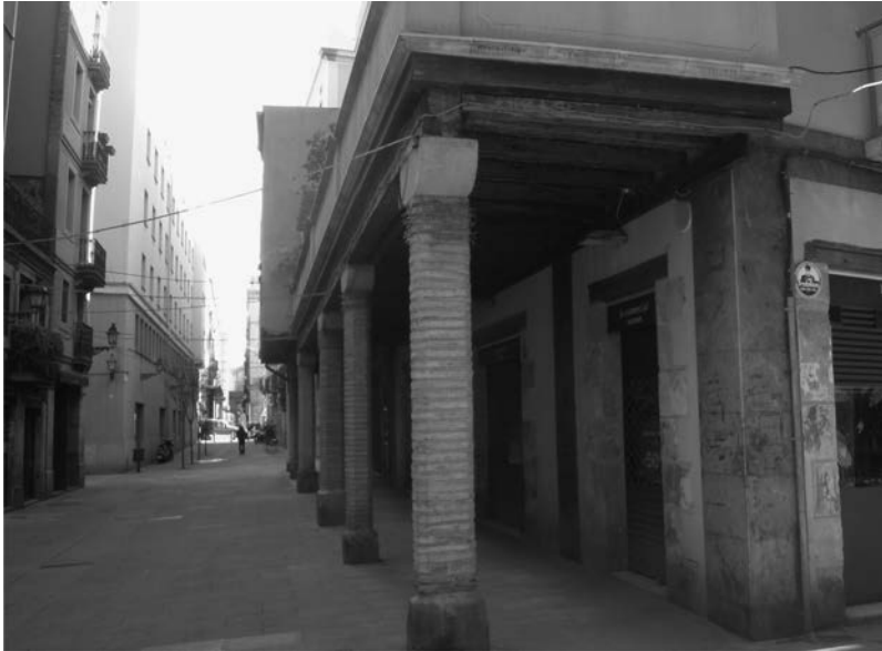
Figure 19.4 The del Rec Comtal street underneath of which the Rec Comtal is flowing (with permission of M. Salgot)
