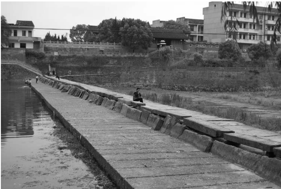
Figure 8.33 Overview of Tashan Weir (Photo taken on 22 May 2011)
