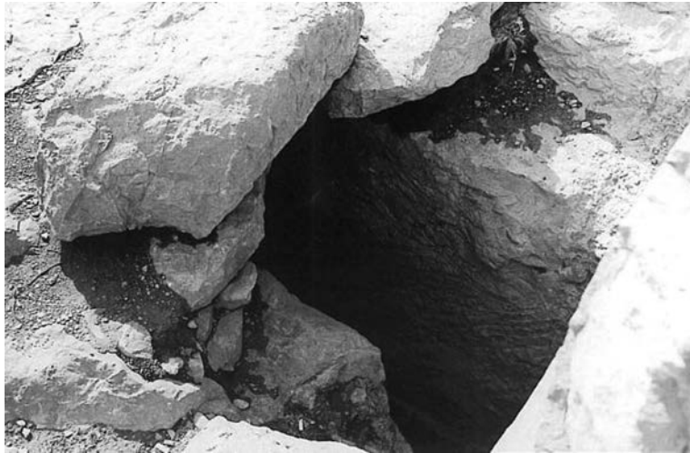
Figure 5.17 Lower segments of the conduits at the sewage outlet
