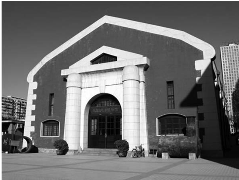
Figure 8.52 Renovated engine room of Beijing Jingshi Waterworks, now Tap Water Museum ( http://www.tour-beijing.com/museums_guide/beijing_museum_of_tap_water.php )
