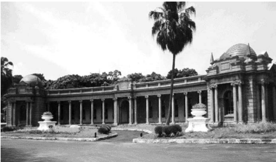
Figure 8.53 Pump Equipment House of Taipei Waterworks of 1908, now Taipei Water Museum ( http://waterpark.twd.gov.tw/english/museum/museum.htm )
