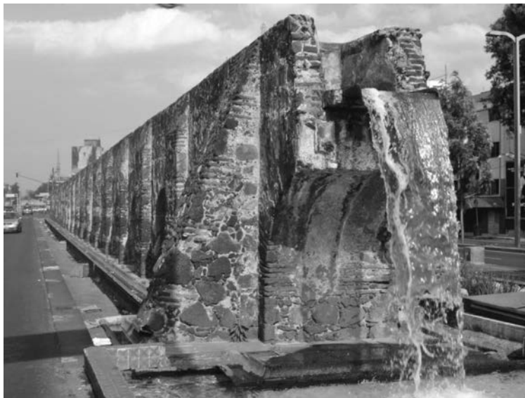
Figure 15.13 Chapultepec aqueduct. Construction of the aqueduct was started in 1620 and completed in 1790, consisting of 904 arches (with permission of Karla S. Estrada Herzfeld)
