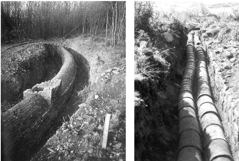
Figure 4.8 Open conduits in Cologne Germany (left). Closed conduits in Pergamos (right) (with permission of G. Karadedos, 2000)
