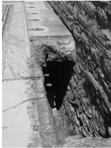
Figure 13.28 Detail of the channel with running water in the latrines in Ephesus
