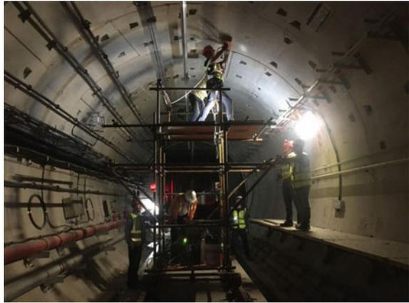
**Fig. 7** Field test photos of seismic wave method
