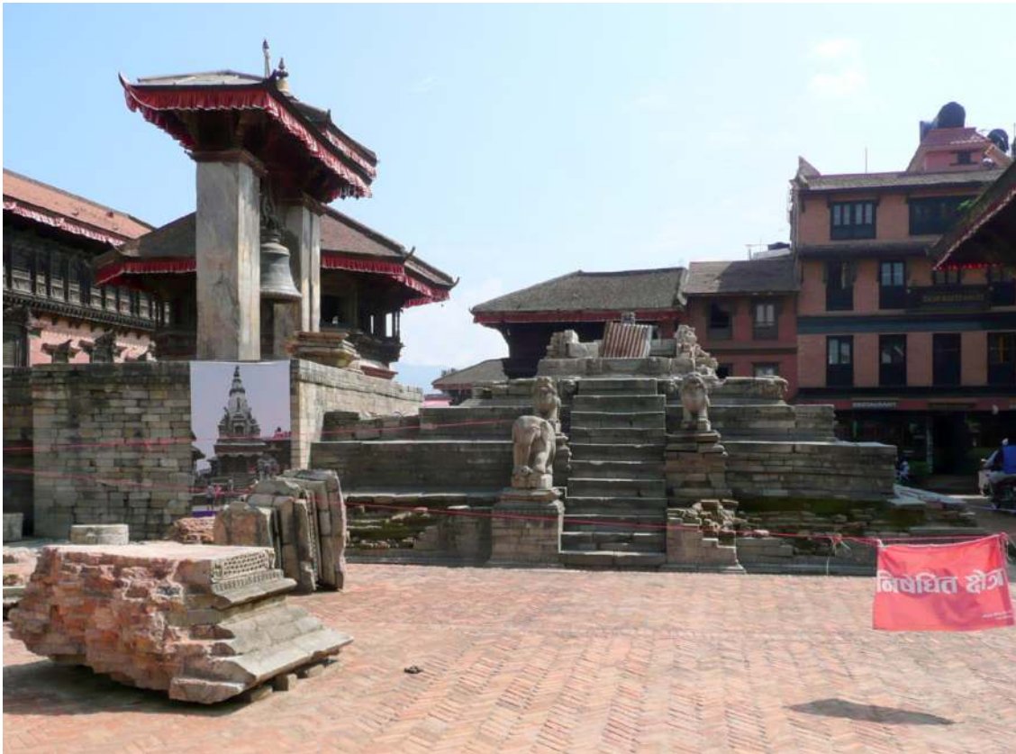
Figure 1. The Vatsala Durga temple (Bhaktapur Durbar Square, Nepal) after its destruction in the 2015 Gorkha earthquakes.
