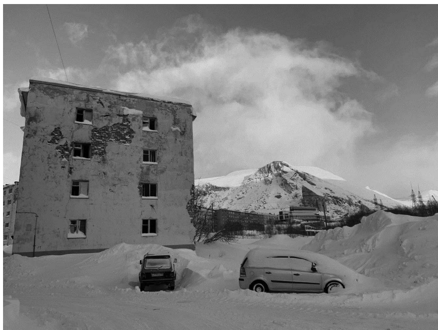
Figure 14.2 Abandoned housing in Kukisvumchorr district of Kirovsk.
