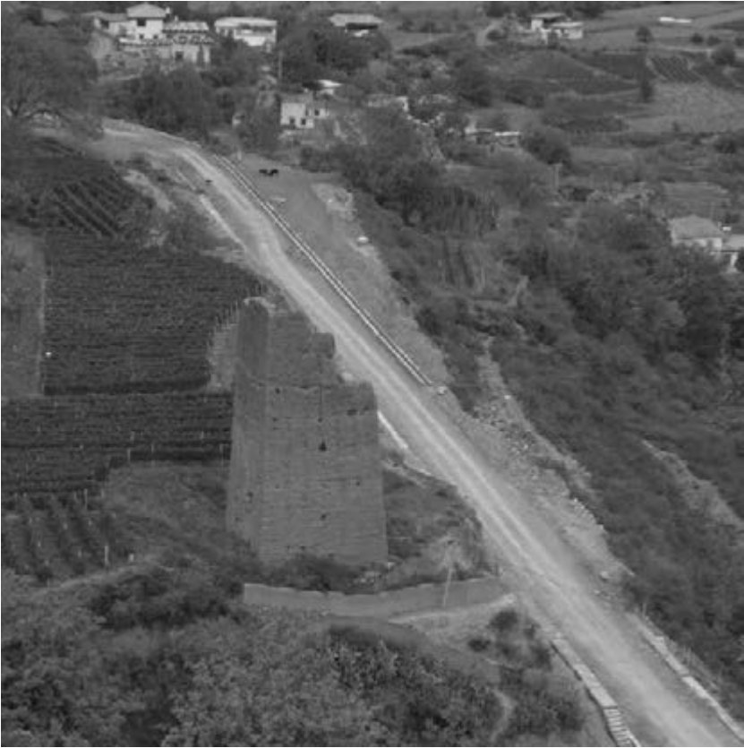
Figure 8.2 Ancient tower, road construction, wine fields, and part of Rongzhong village
