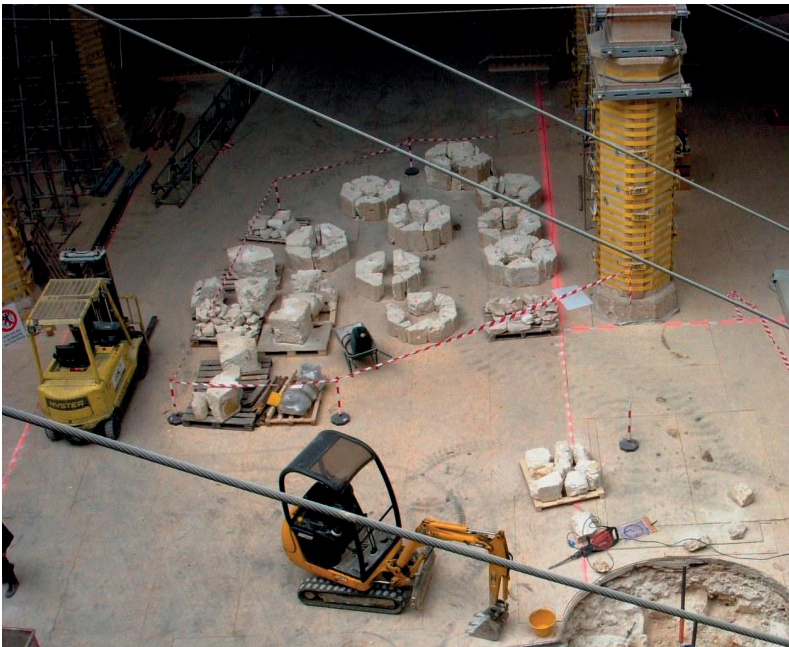
Figure 1.4 Santa Maria di Collemaggio: the dismantled pillars during the restoration works.
