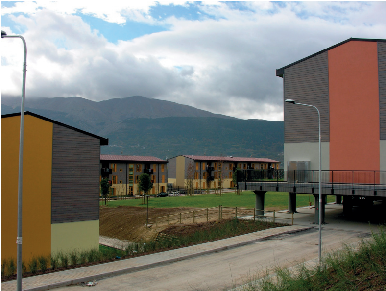
Figure 5.11 View of the CASE in Bazzano in 2015. The buildings rest on seismic-reinforced concrete plates, supported on metal pillars fixed to a foundation, also of reinforced concrete. Photo: Vincenzo Di Florio.
