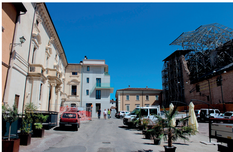
Figure 5.4 L’Aquila: Piazza Paganica in July 2020 – on the left is Palazzo Ardinghelli, location of MAXXI L’Aquila, on the right, the Santa Maria church. Photo: Francesco Giancola.
