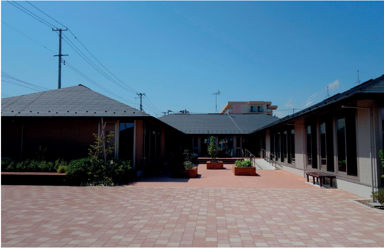
Figure 3.6 The exterior of the collective-type public housing for mutual assistance in Ishinomaki.
