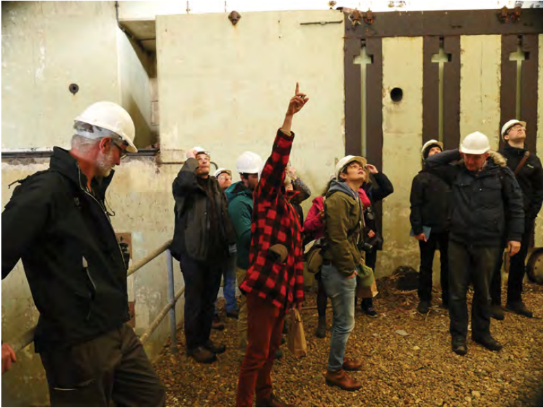
Figure 23.3 Workshop participants inside one of the AWRE laboratory buildings observing decay (photograph by Antony Lyons).
