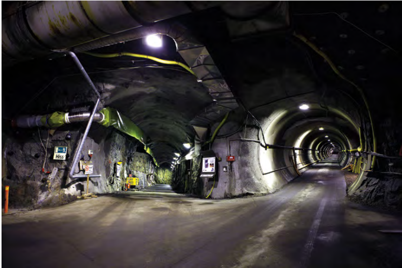
Figure 2.1 Part of the network of tunnels at SKB’s Final Repository for Short-Lived Radioactive Waste located at Forsmark in the municipality of Östhammar (photograph courtesy of SKB).
