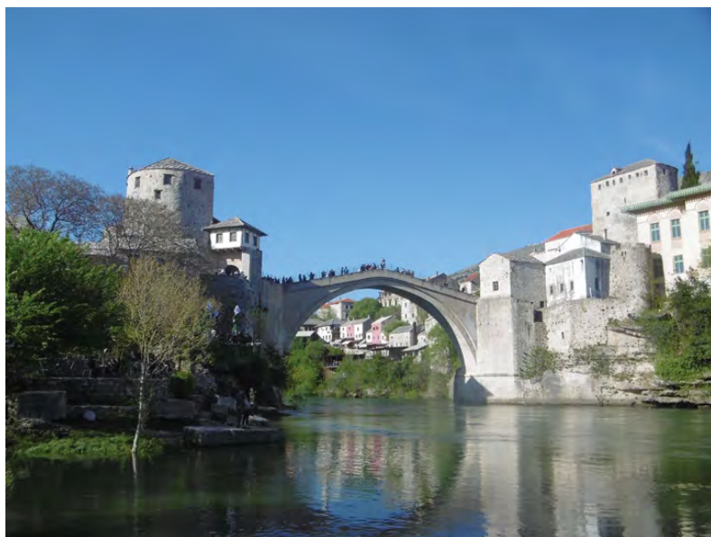
Figure 19.5 The reconstructed Stari Most bridge in Mostar, Bosnia and Herzegovina (photograph by Gustav Wollentz).
