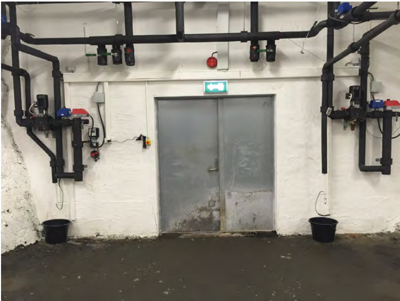
Figure 5.15 Entrance to one of the three identical refrigerated storage recesses inside the Svalbard Global Seed Vault (photograph by Rodney Harrison).
