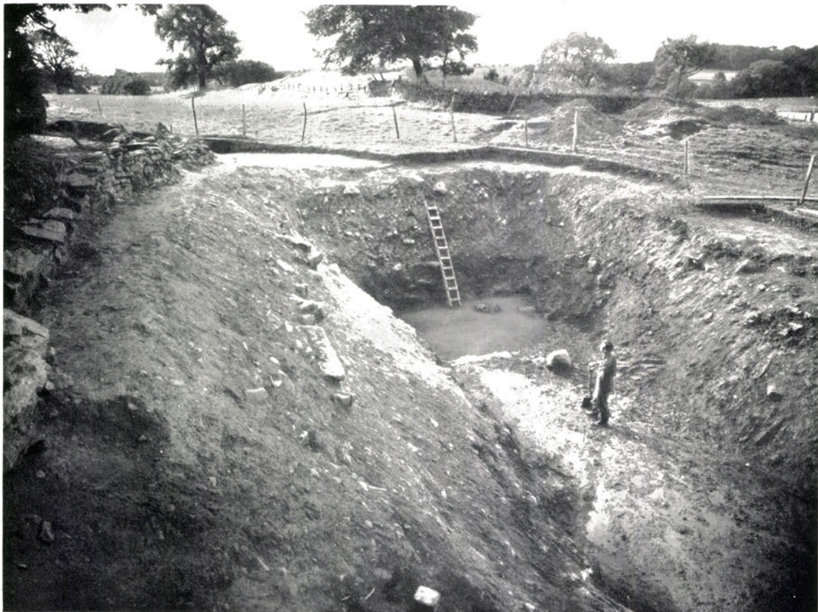
b. Phase II, Site B, showing a 50-ft. stretch of the ditch cleared. The man stands on the rock-cut bottom of the ditch; the ladder leans against the solid causeway at the end of the ditch. On the left is the base of the stone-revetment. The sword, &c., were found in the pool at the end
