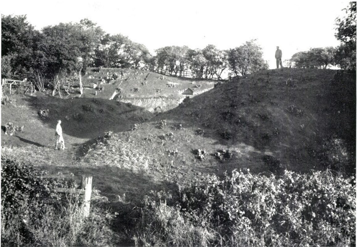
b. The same after preliminary clearing. The right-hand figure stands on the salient or bastion; the left-hand figure marks the present level of the ditch; beyond the bastion the sun lights the intended position of the gate
