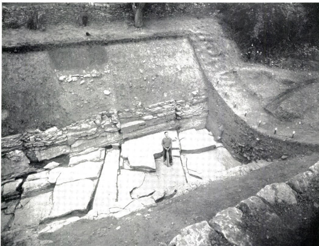
b. Phase II, Site A, view of the rock-cut ditch from the summit of the rampart. In the right foreground is the edge of the rebuilt revetment
