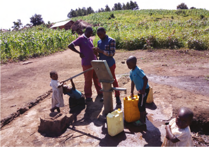
Figure 9.8. This (Formal) Public Amenity – a borehole with handpump ('Bush Pump') would be 'coded' in OpenStreetMap with the conventions of Key and Tag respectively. In this instance, 'man_made' = 'water_well', and 'pump' = 'yes'.
