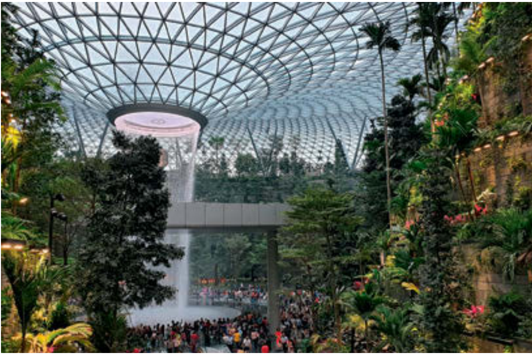
226 Singapore, Changi Airport, glass-domed 10-storey mall extension (2019) with 40-metre-high waterfall.
