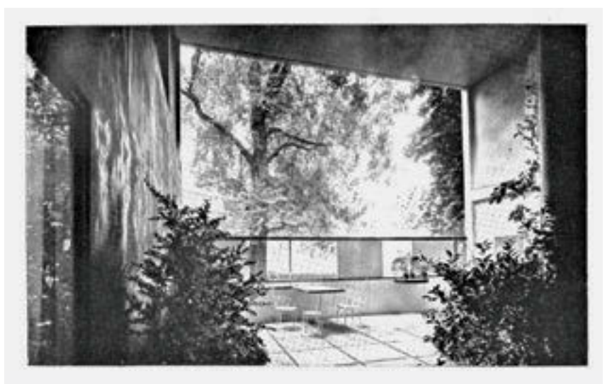
47 Le Corbusier, Pavillon de l'Esprit Nouveau, simulating the vista of future high-rise buildings, Paris 1925.
