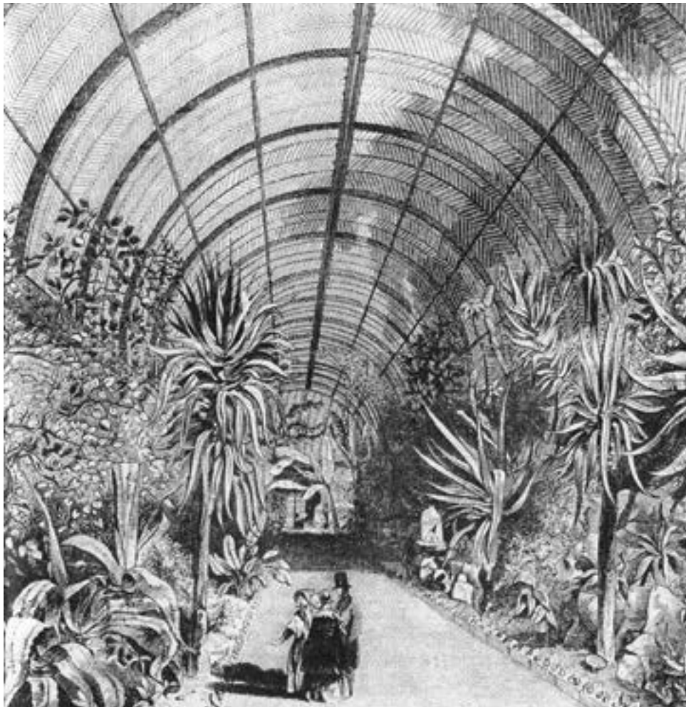
6 Joseph Paxton, Conservatory (84m long, 37m wide and 19m high) in Chatsworth (UK), 1840.
