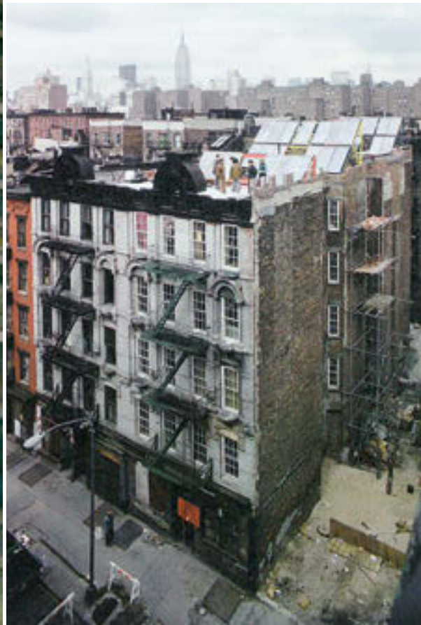
203 Early initiative in decentralizing the energy supply by using urban climatic forces: Solar collectors and a windmill installed by the residents, Lower East Side, New York, 1976.
