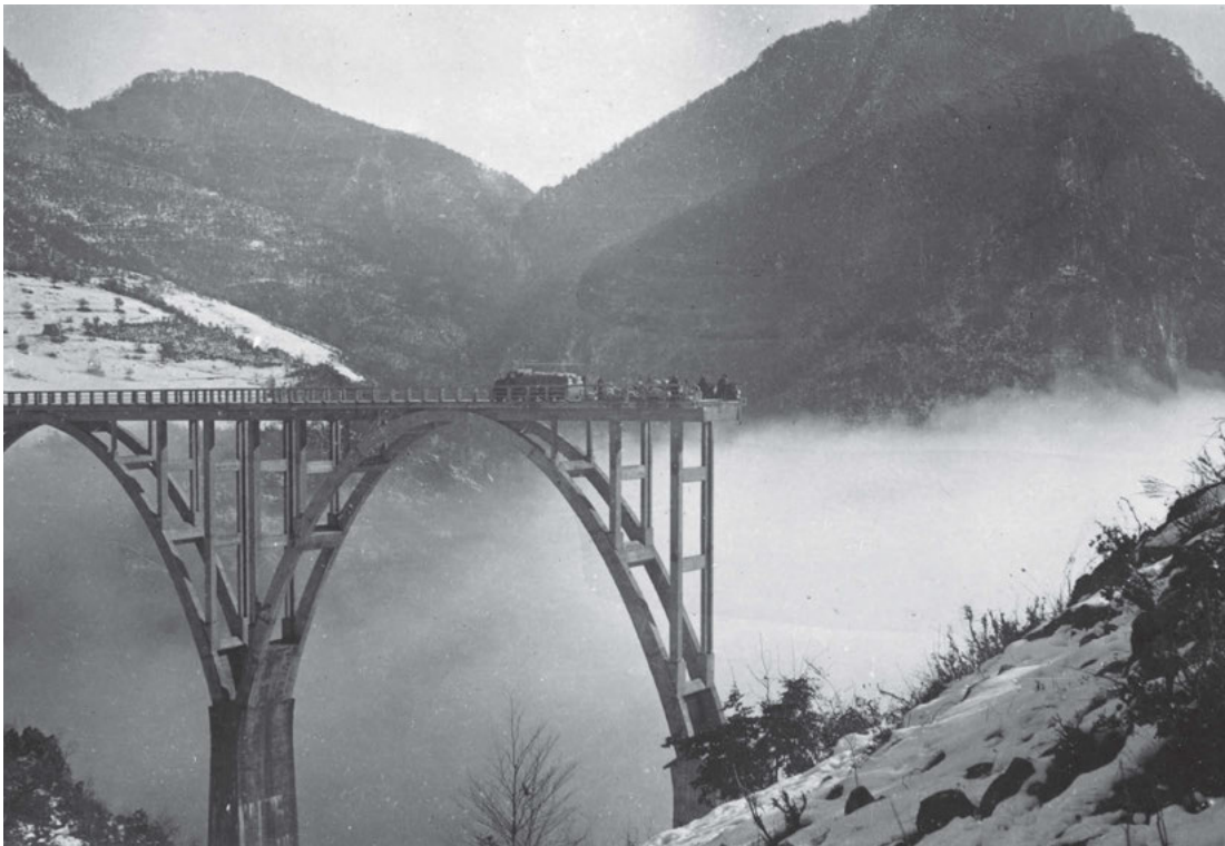
Destroyed bridge on the river Tara, Montenegro, 1943. Croatian History Museum, HPM-MRNH-F-1043.
