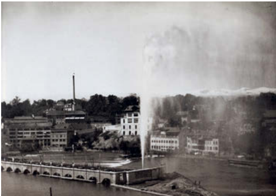
17 The hydro plant of Forces Motrices (as yet, without its turbine hall) releasing residual pressure every evening via a safety valve, hence being the main attraction in the city, c. 1886.
