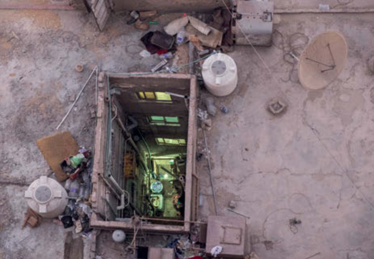
103 Light-well ( manwar ), a common architectural feature supposed to allow the ventilation of the rooms that have no direct access to the exterior.
