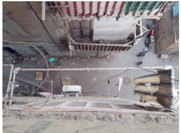
104 Shreds of curtain remained hanging on curtain rods attached to the front of Umm Rania's building.
