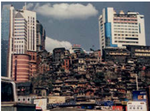
77 Old postcard of stilted houses next to high-rises in Caiyuanba , probably 1990s.
