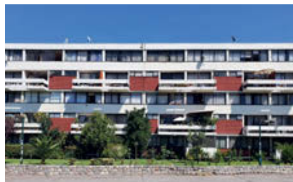
51 Villa Frei , façade of a "Duplex block."
