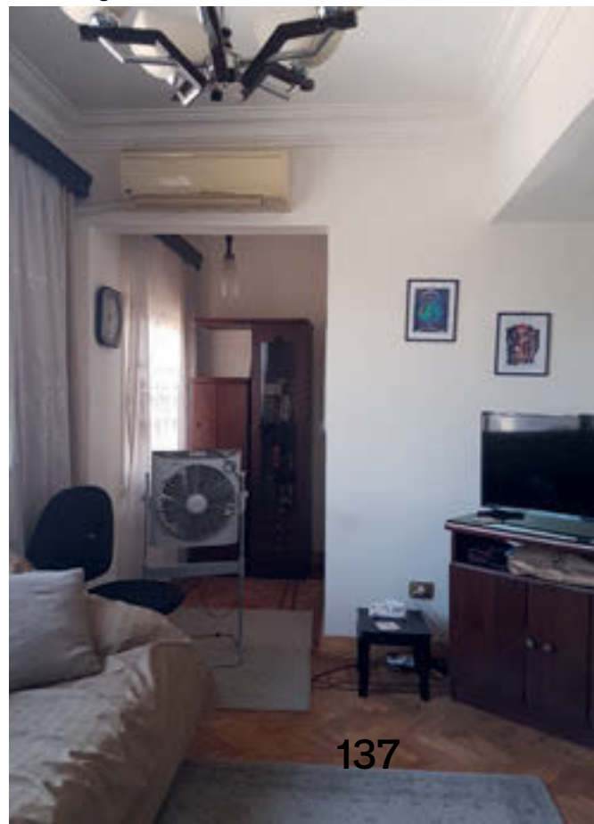
111 The "greenhouse" in Magda's apartment. The sun hitting the steel roof heats the room in the background nicely in winter, but is more constraining in summer.
