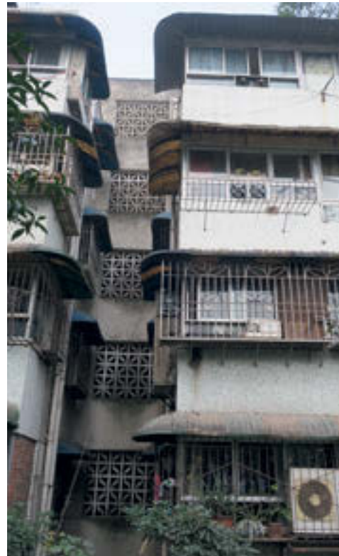
81 Xiao Meishu Xueyuan , side façade of an apart- ment house from the early 1990s. Note the staircase built with “ventilation bricks” ( tongfeng zhuan ), rain protection above the windows, and the self- installed window and split- unit air-conditioners.
