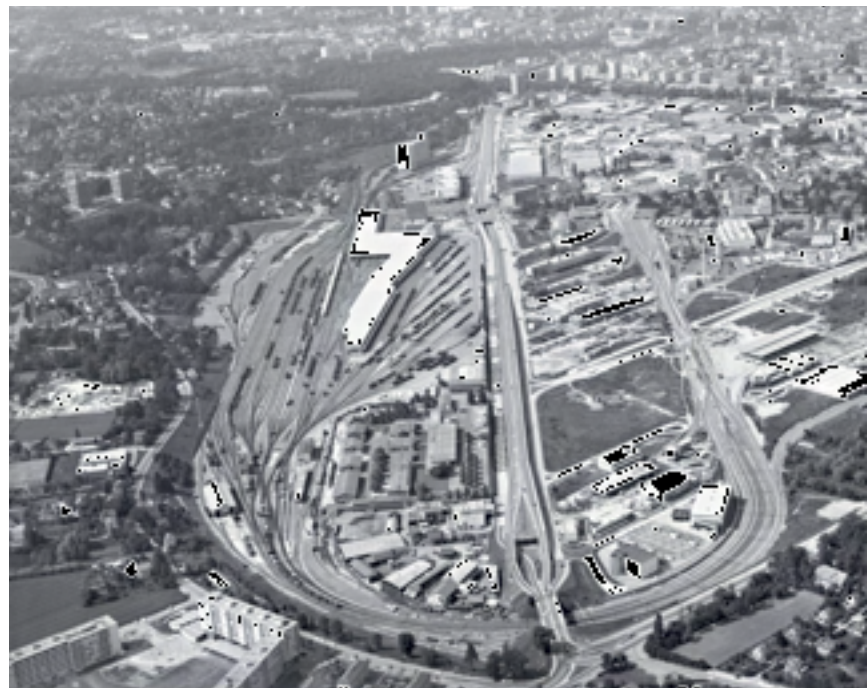
31 The steady transformation from an alluvial plain into a transport-infrastructure hub for cargo handling, here seen in 1968.
