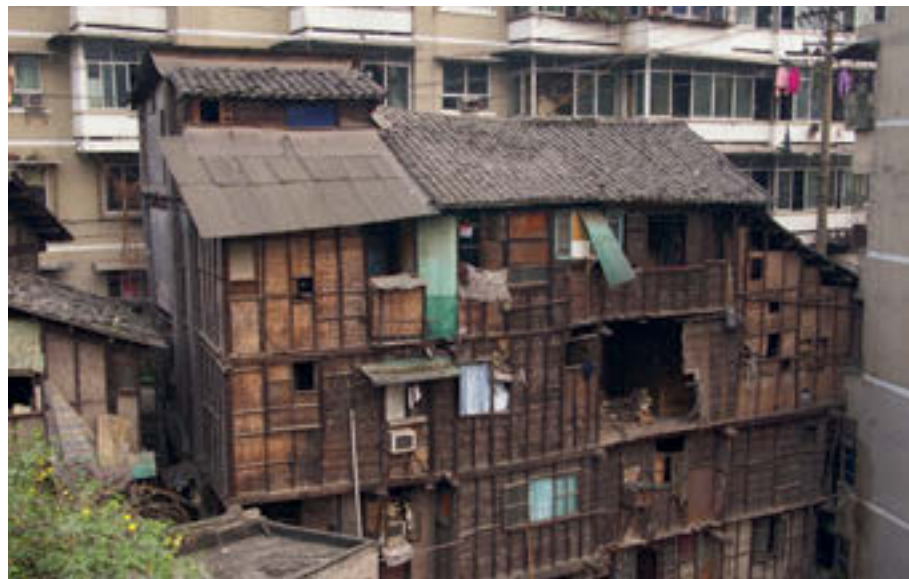
78 An old wooden-stilted building in Shibati neighbourhood in 2010 surrounded by modern apartment buildings. Note the “breathable” bamboo walls.
