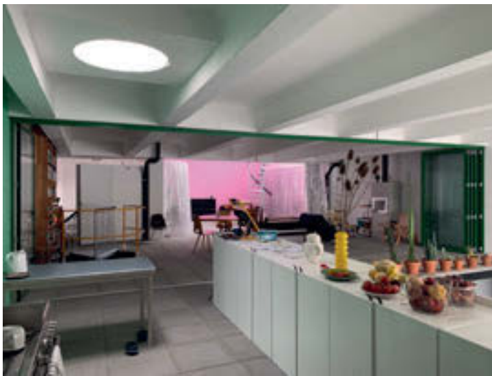
36 The adaptable element of the folding door serves as architectural tool of thermal control. View of the kitchen area with its sky window.
