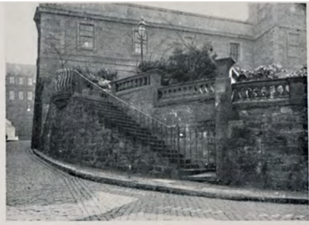
FIG. 7. — The same entrance, showing effect of lowering and balustrading wall, and exposing staircase with shrubbery above. A simple example of detail of formal gardening applicable to varying levels.
