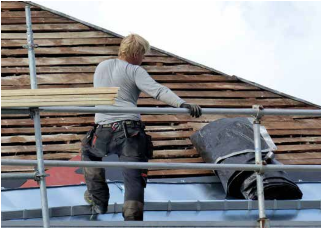
↻ Repair of a roof with a wooden board in old Rauma, Finland (© F. Vegas, C. Mileto, 2017)
