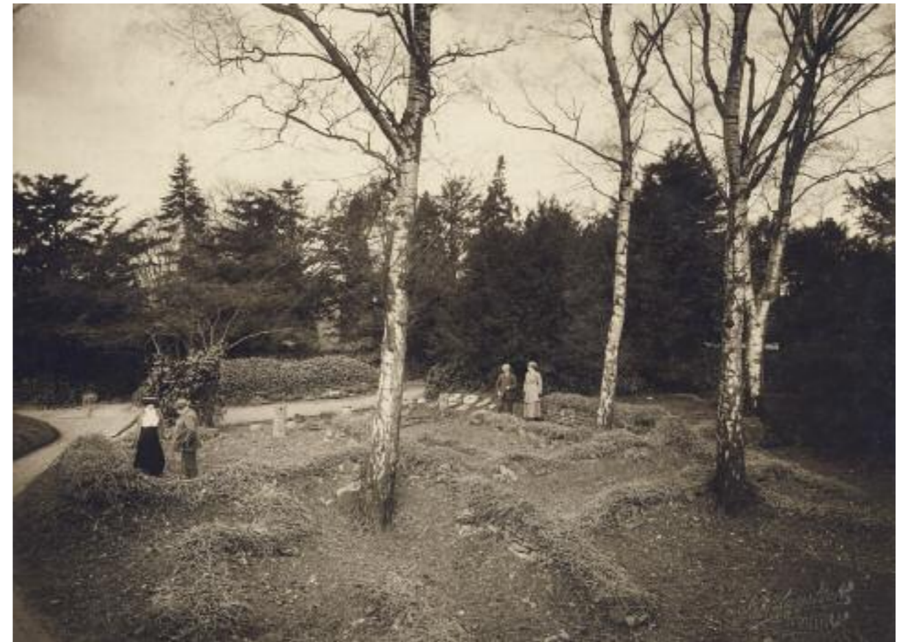
Fig 1.5 Photograph of an excavated Roman building (G10) and architectural fragments displayed in the garden of Aldborough Manor, c 1910. The Roman Town Wall (G9) lies just beyond the path, covered in ivy. Viewed from the west. Photograph: T J Hanstock. Reproduced by courtesy of Sir Andrew Lawson-Tancred
