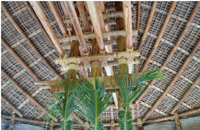
Figure 7.2: ’Afa binding on the roof structures in the fale at the Tiapapata Art Centre, Apia, 2014. Photo: Steven Percival.
