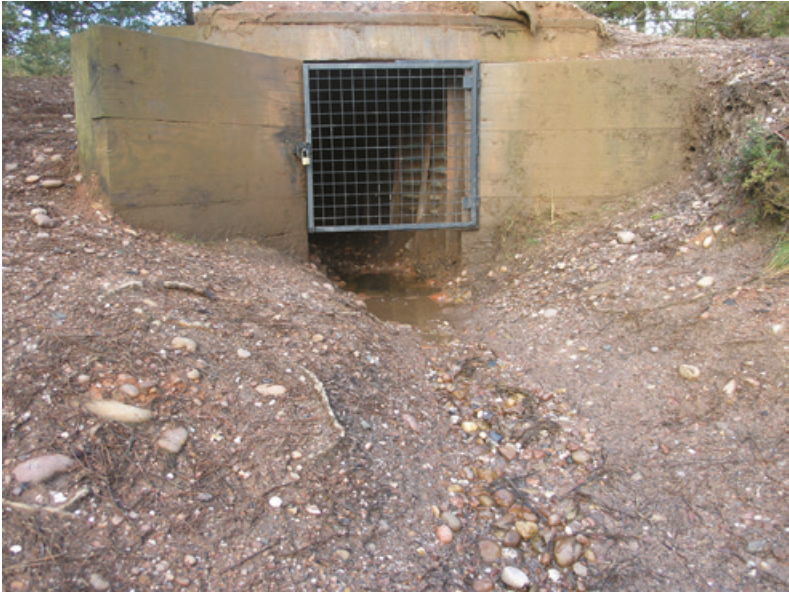
Figure 3.9A Exit of dry tunnel
