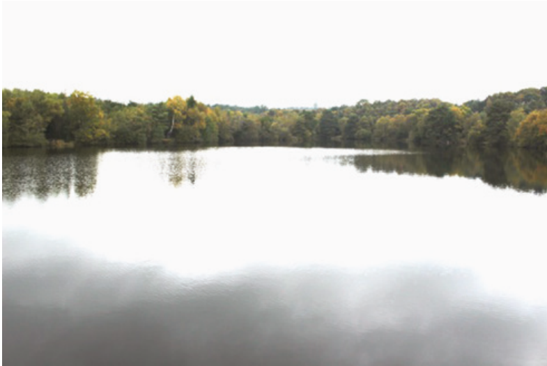
Figure 10.1 Squabmoor reservoir looking north
