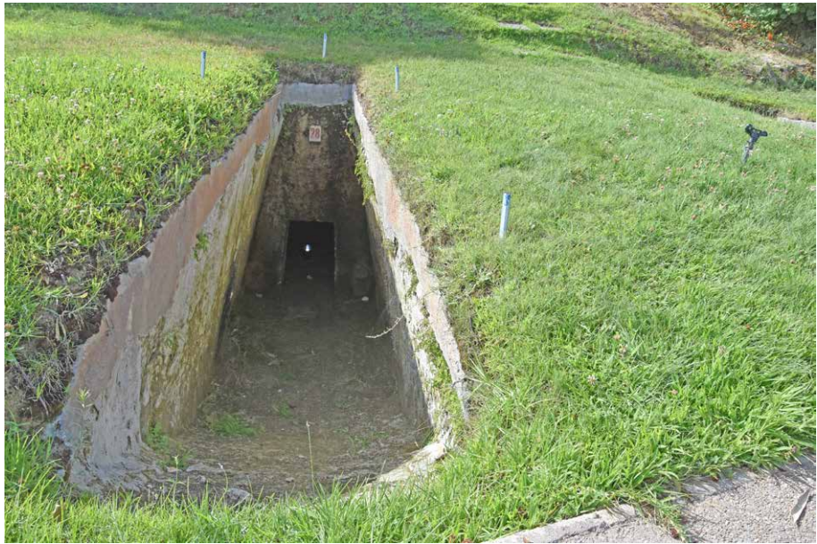
Figure 4.3.16. VT28 entrance, facing south-southeast.
