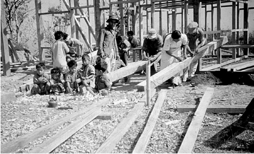
FIGURE 9.5 Communal labor. Planing planks for a new clinic in Pukzing village, 1956. PHOTOGRAPHER UNKNOWN (POSSIBLY GWEN REES ROBERTS). REPRODUCED BY PERMISSION OF AIZAWL THEOLOGICAL COLLEGE COLLECTION, AIZAWL, MIZORAM, INDIA
