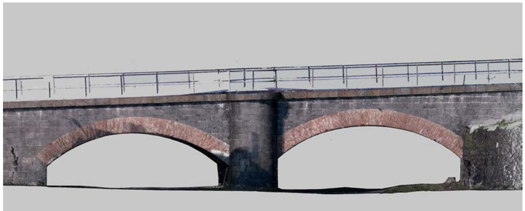
Orthophoto of the two-arches bridge on the Birbo stream (Piedimonte, Catania).
