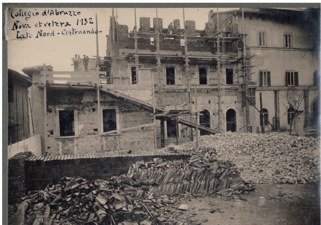
Fig. 4. Historical photo of the construction site of the north part of the building.
