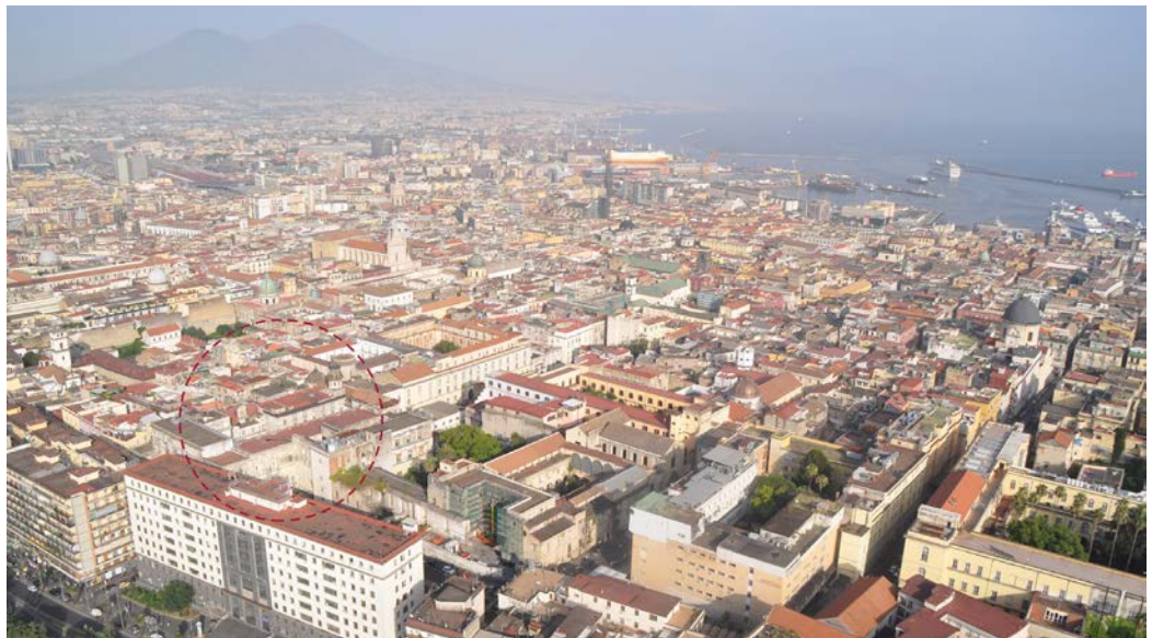
Fig. 1. Survey by the Benecon airborne platform, view of the City of Naples and focus on the Historic Pharmacy of S. Maria del Popolo degli Incurabili.
