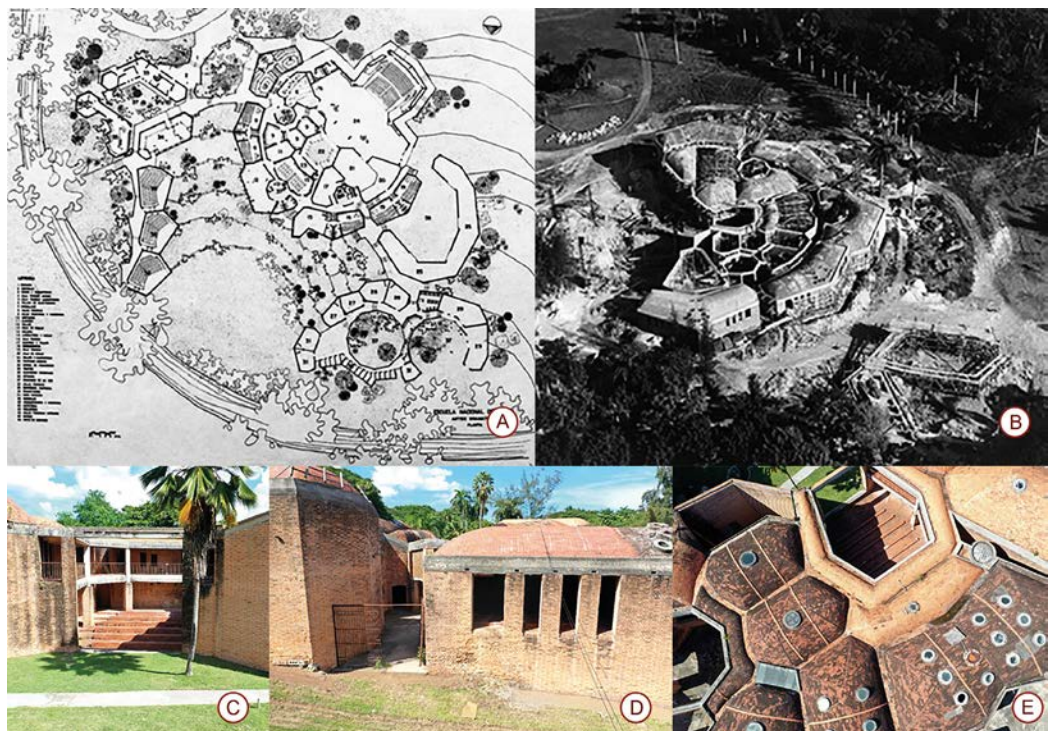
Fig. 1. In order from left to right: original design plan (a), site photos (b), view of the interior courtyard from the main access (c), exterior view of a portion of the complex (d), aerial view of the roof system with tabicadas vaults (e).
