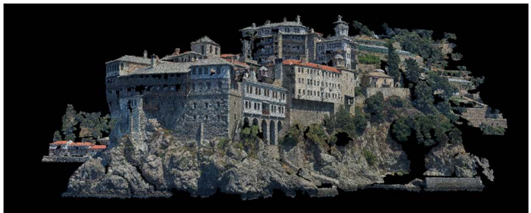
The Monastery of San Gregorio. Cloud of points made from the sea.
