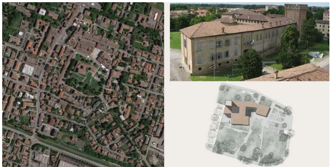
Fig. 1. Aerial and photographic images of the Rocca of San Martino in Rio; bottom right, the plan of the roofs of the building with the drawing of the public park that surrounds it.
