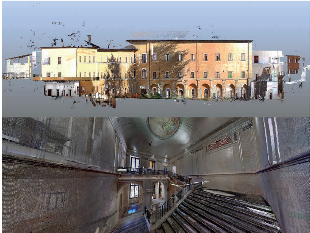
Fig. 2. 3D surveying: The courtyard facades, and the monumental staircase.
