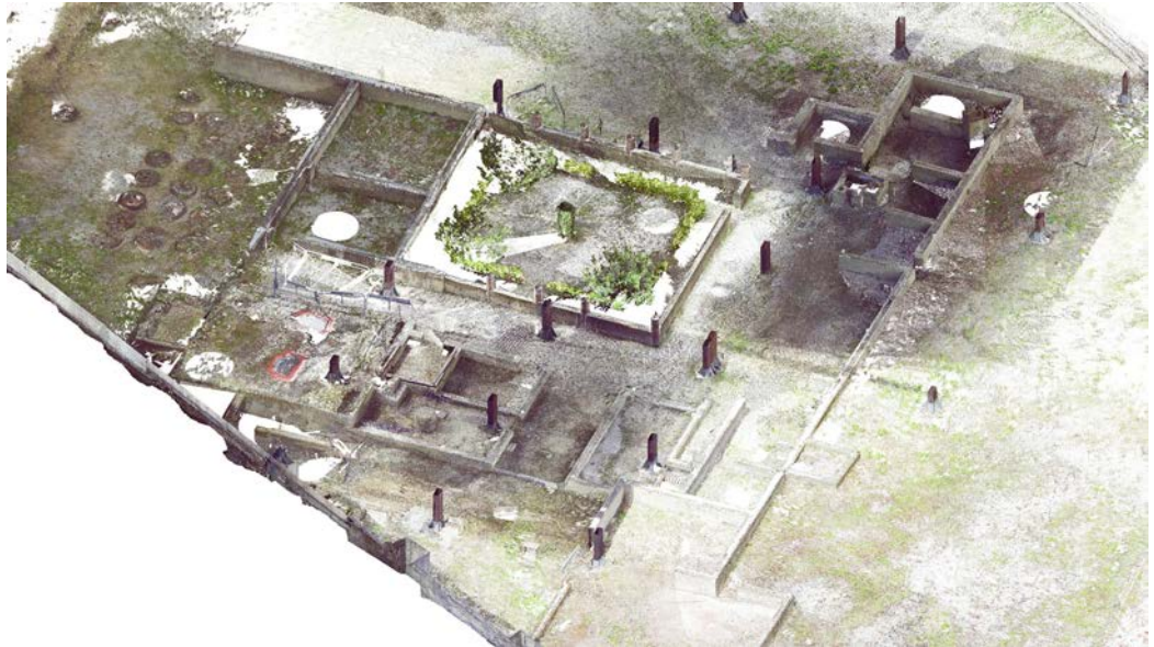
Fig. 7. Point cloud of the villa obtained by processing of the survey data.
