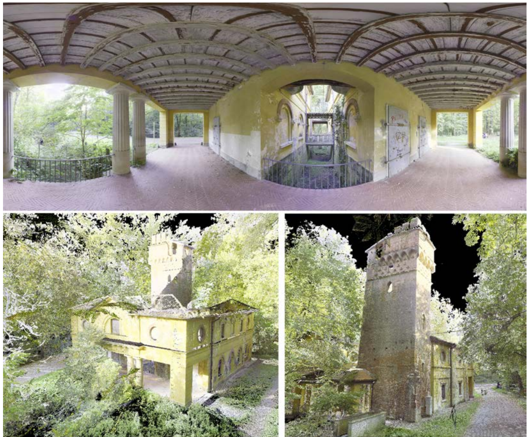
Fig. 3. Spherical image captured by TLS station n. 7 (on the bottom) and the perspective view from the Southeast (on the left) and Northwest (on the right) corner of the final colored point cloud formed by the aligned scans.
