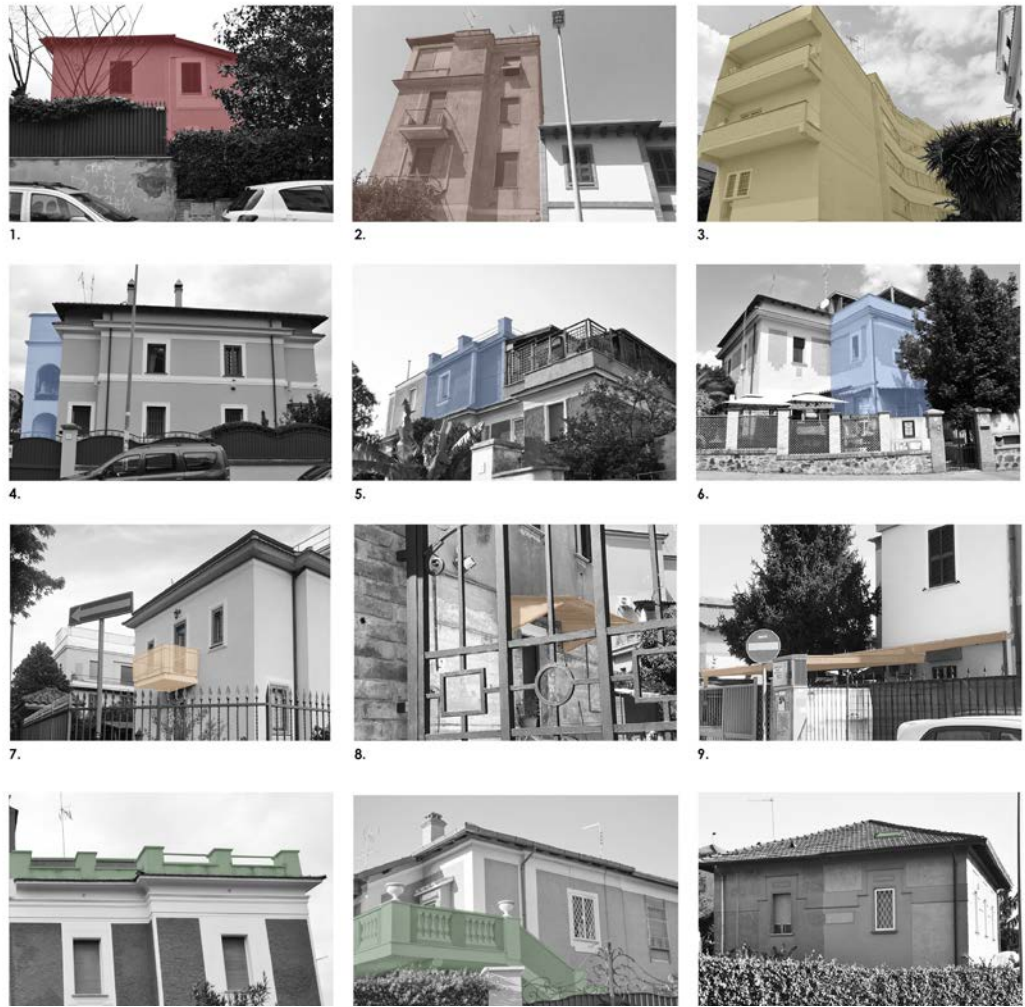
Fig. 10. Photomosaic of the main building modifications of the villini in the garden borough of Pigneto (graphic elaboration by V. Apostoli).
