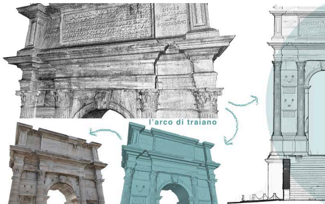
Fig. 9. Three-dimensional in-depth study of Trajan's Arch, one of the POI of the Local Virtual Museum of Ancona seaport. Point cloud, mesh model, textured model, and grayscale orthoimage.
