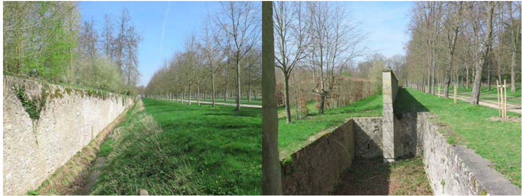
Fig. 6. The Petit Trianon Park of Versailles, the Ah-Ah device used to define the south-eastern boundary, view (photo by D. Crispino, 2017).
