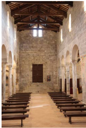
Fig. 4. Main façade with entrance stairs seen from within.
