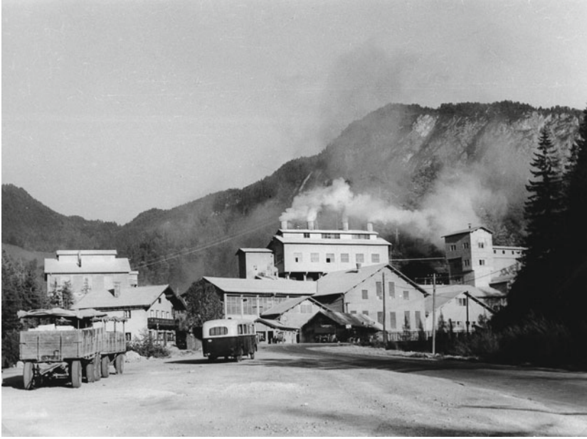
Fig. 7.5 The cement plant seen from the entrance on the Eibergerstraße, 1962. The four shaft kilns are clearly visible in the background
