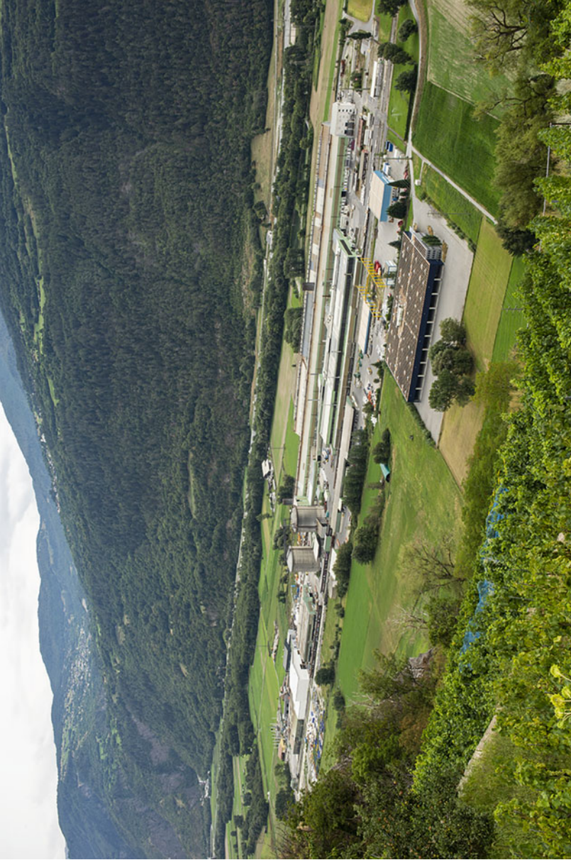
Fig. 7.86 Overview of the former aluminium smelter, which lays in the centre of the Rhone valley bed surrounded by monocultures
