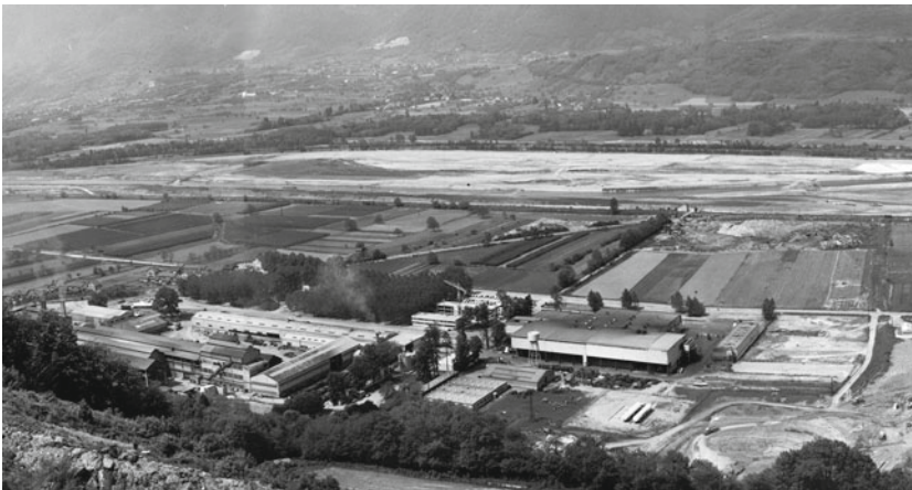
Fig. 7.33 Overview of the expanding industrial site from the Brame Farine slopes, in 1974. In the background, the EDF basin being created
