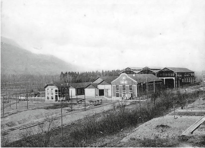
Fig. 7.31 The steelworks in the first years of activity, around mid 1920 s
