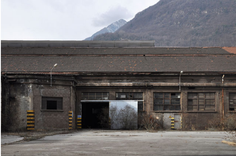
Fig. 3.5 Empty halls of the former SISMA steelworks in Villadossola, 2016
