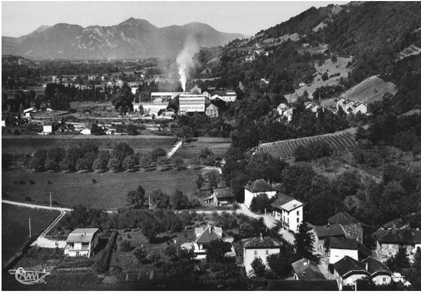
Fig. 7.32 The steelworks and the attached workers settlements, immersed into the agricultural landscape of the upper Gresivaudan, ca. 1950
