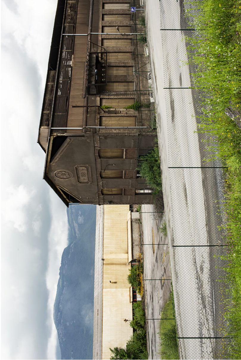
Fig. 7.41 The oldest existing building on the site (dating back to 1921, as written on the facade), a former power substation
