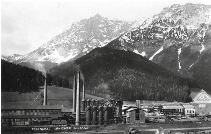
Fig. 3.2 The ÖAMG blast furnaces in Eisenerz, 1921
