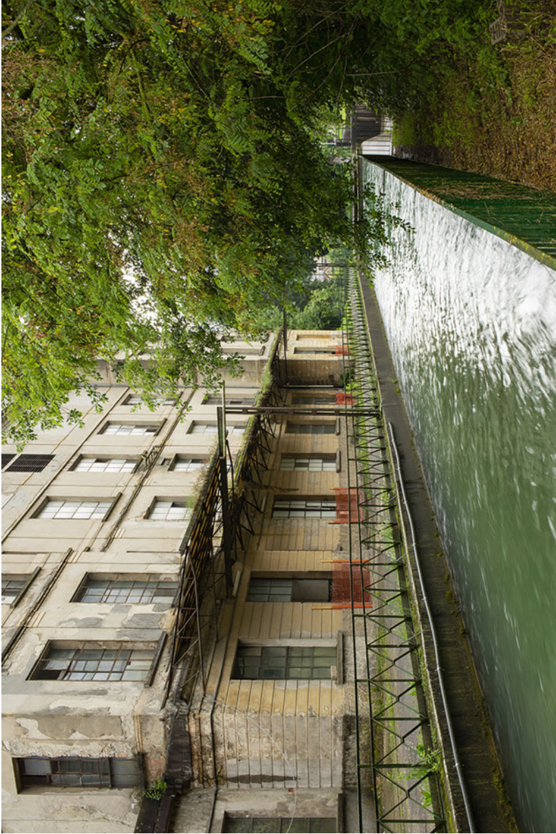
Fig. 7.70 The hydropower canal runs through the entire site to bring water to the power station and production halls. On the left, the imposing new spinning mill
