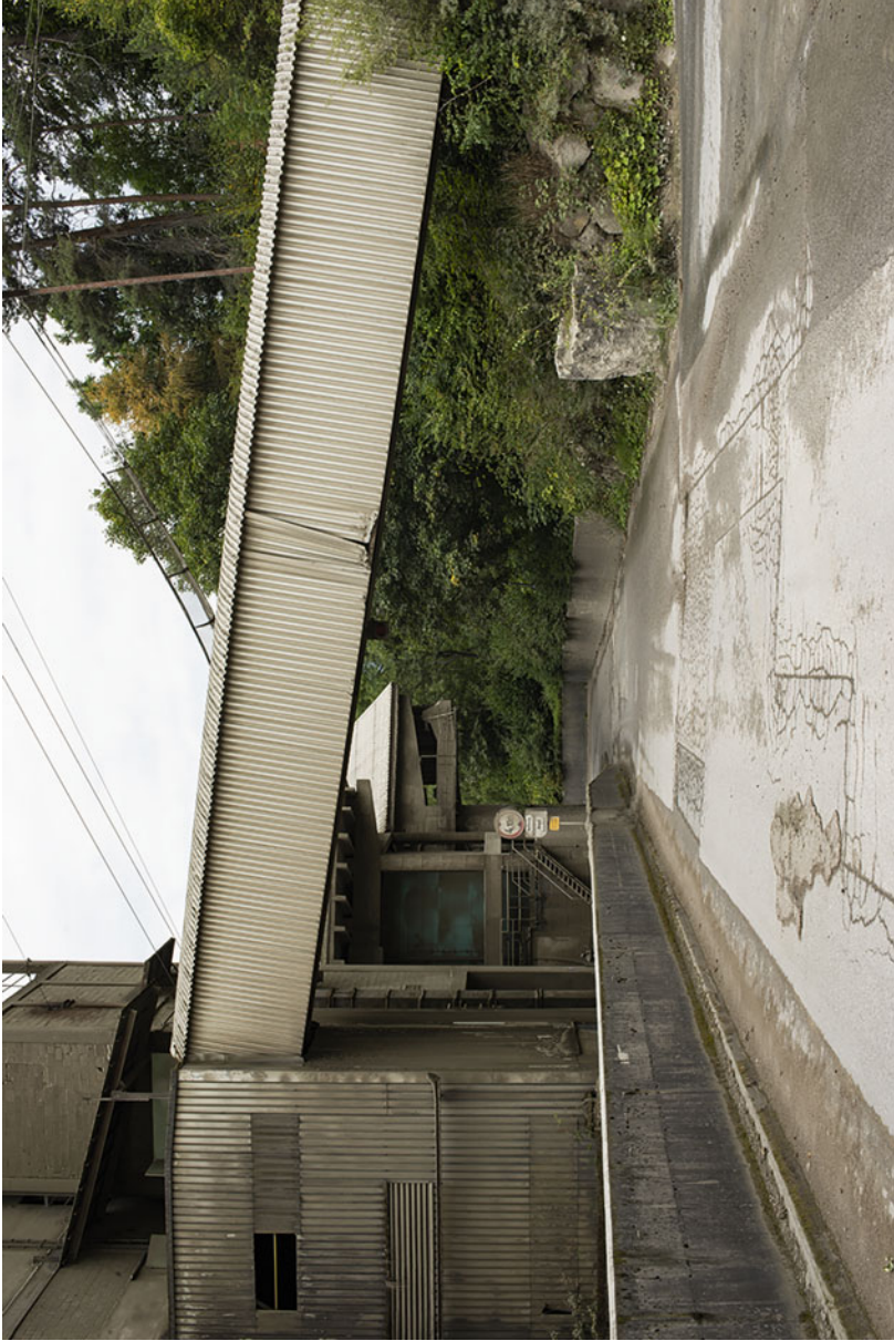
Fig. 7.16 An aerial conveyor belt connecting the disused production halls to the clinker silo
