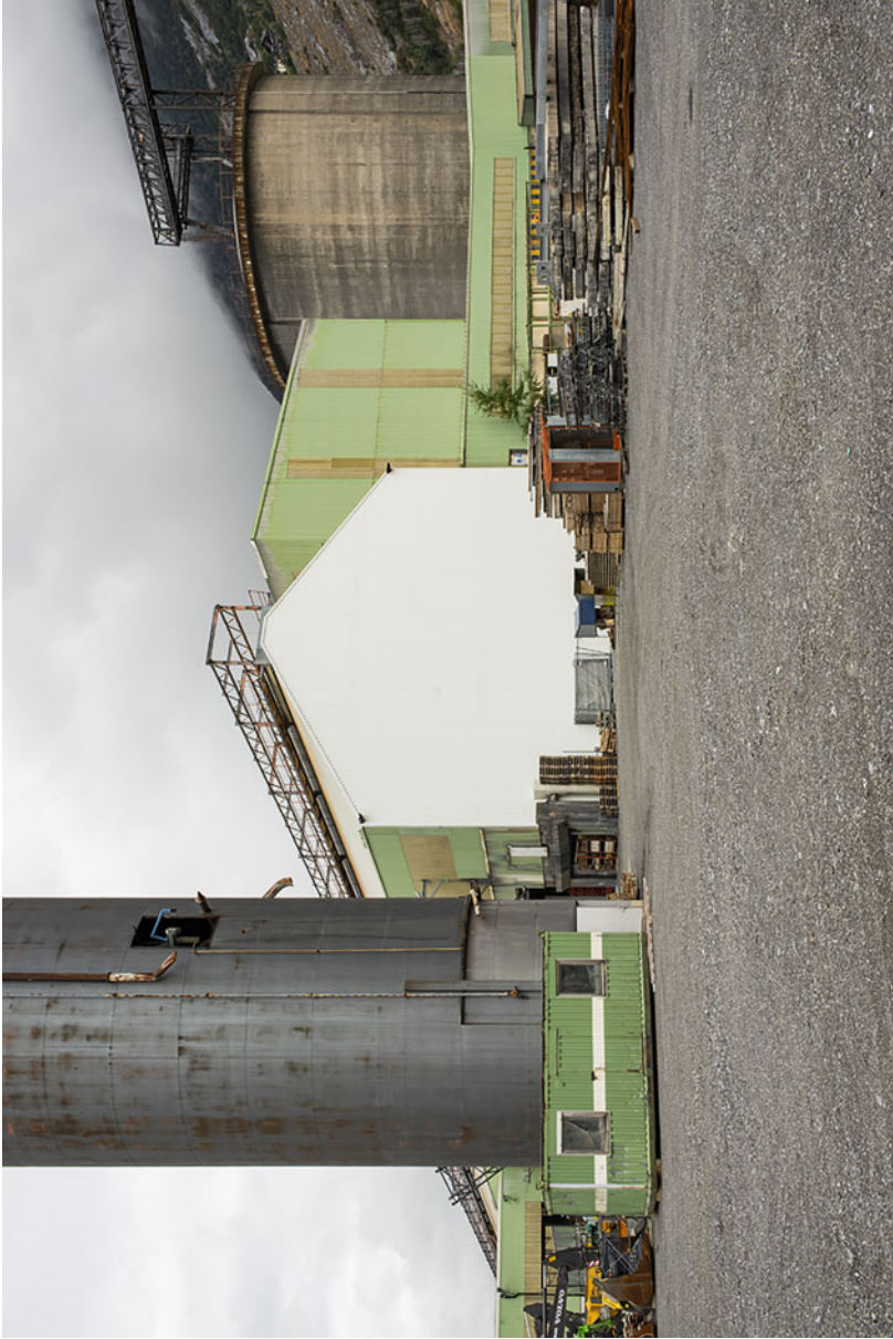
Fig. 7.94 A large concrete apron (owned by Theler AG) surrounded by former industrial objects. Left to right: a gas washing tower, the first electrolysis hall and the alumina silo
