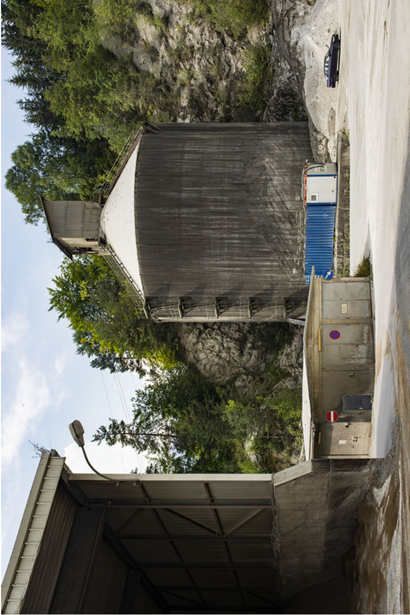
Fig. 7.17 The massive clinker silo standing next to the bare rocks in the ancient Haberg quarry site
