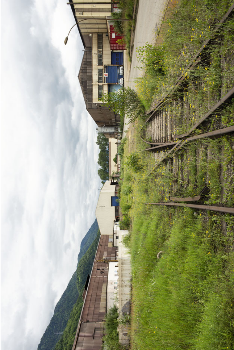
Fig. 7.46 Abandoned railway tracks running south, flanked by the two rolling mills
