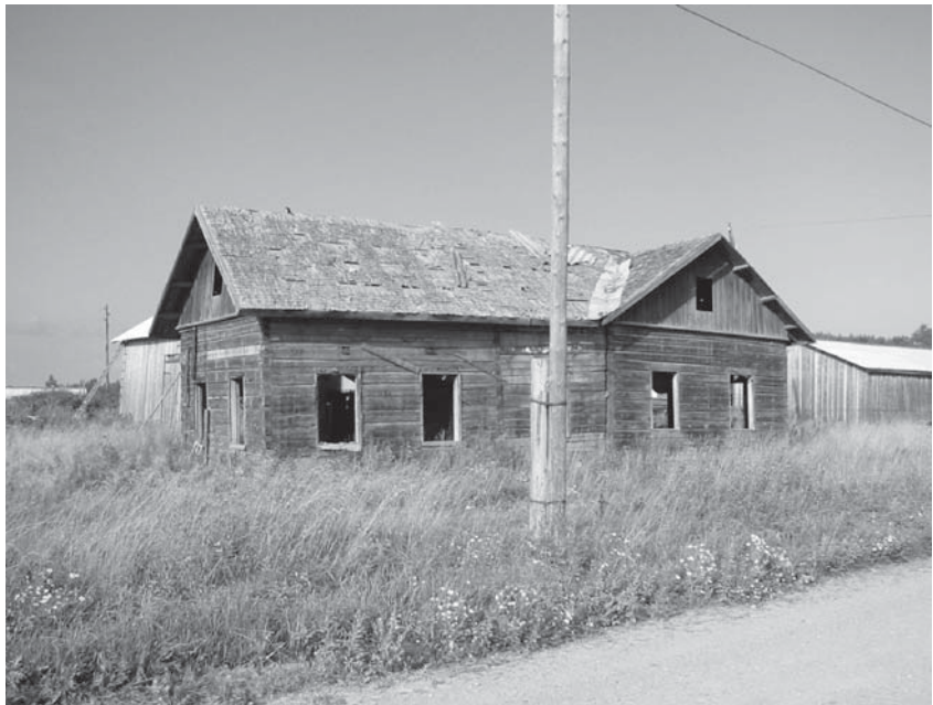
A Finnish house partially dismantled and the timber numbered for transportation purposes. Kurkijoki 2002. (Photo: Pekka Hakamies)
