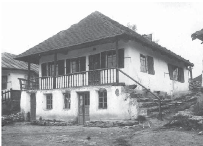
House in Shargorod (late 19th century). Since 1922 till 1942 this building was owned by Moshe Shaevich Reifman. Photo of 1930s. Personal archive of A. Sokolova. In this photo one can see the front door entrance which led from the gallery to the hall. (Photo: A. Sokolova)
