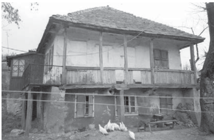
Empty Jewish house in Sharhorod. The building is in an emergency condition. (Photo: A. Sokolova 1993)
