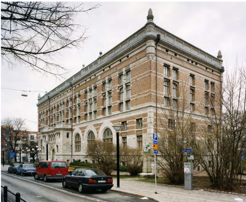
Figure 5.2 City and university library from 1901, reopened as university library in the 1990s after a period as city archive. In a park but not withdrawn from the street. Photo: Krister Engström
