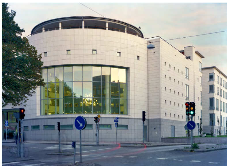
Figure 5.7 School of Economics from early 1990s in a block of its own next to the faculty of social sciences. On the corner the library with a large ‘urban window’. Photo: Krister Engström
