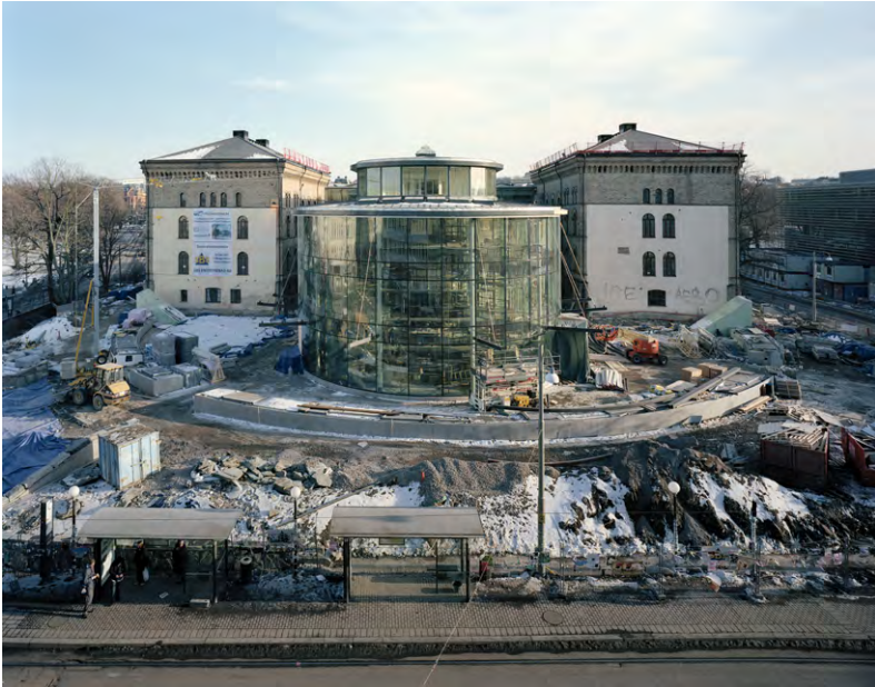
Figure 5.5 New faculty of Education, built in 2006 as an addition to an 1850s hospital. The only externally located faculty now became the only one inside the moat of the former fortifications. Photo: Krister Engström
