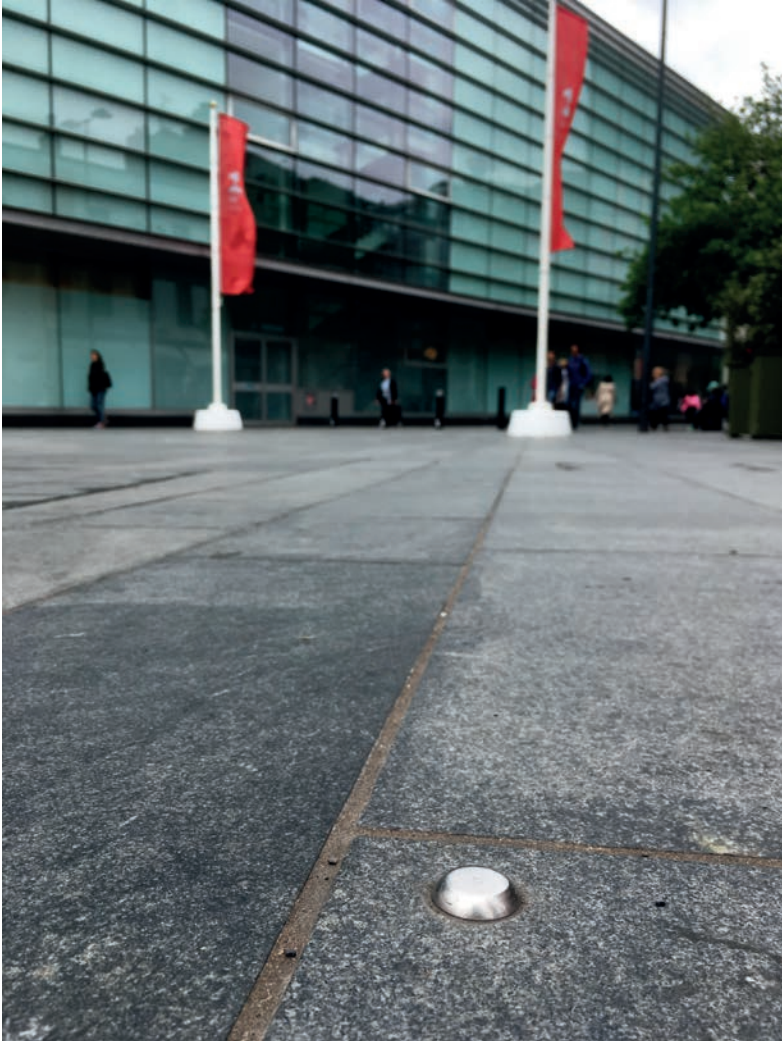
Figure 1.3: Liverpool ONE: metal studs reveal the legal boundary, and are not always situated at the branding boundary. © David Littlefield
