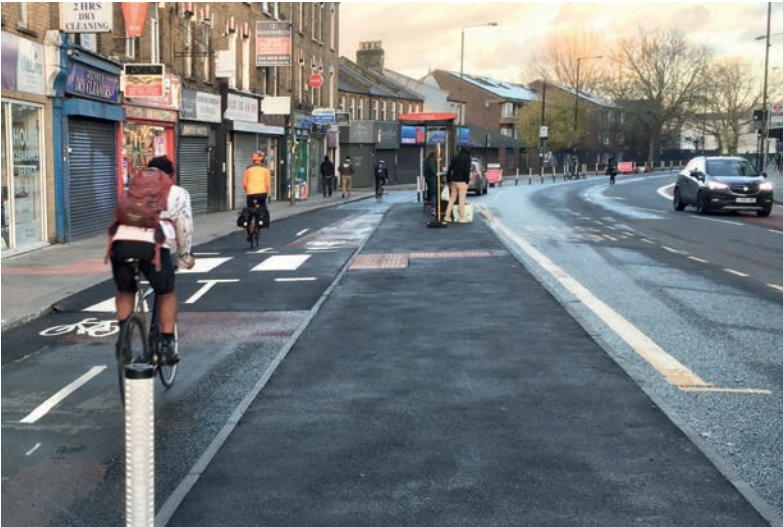
Figure 13.7: New cycle lanes, re-prioritising street space permanently in East Greenwich (one of the unimproved Street Appeal case studies). © Matthew Carmona
