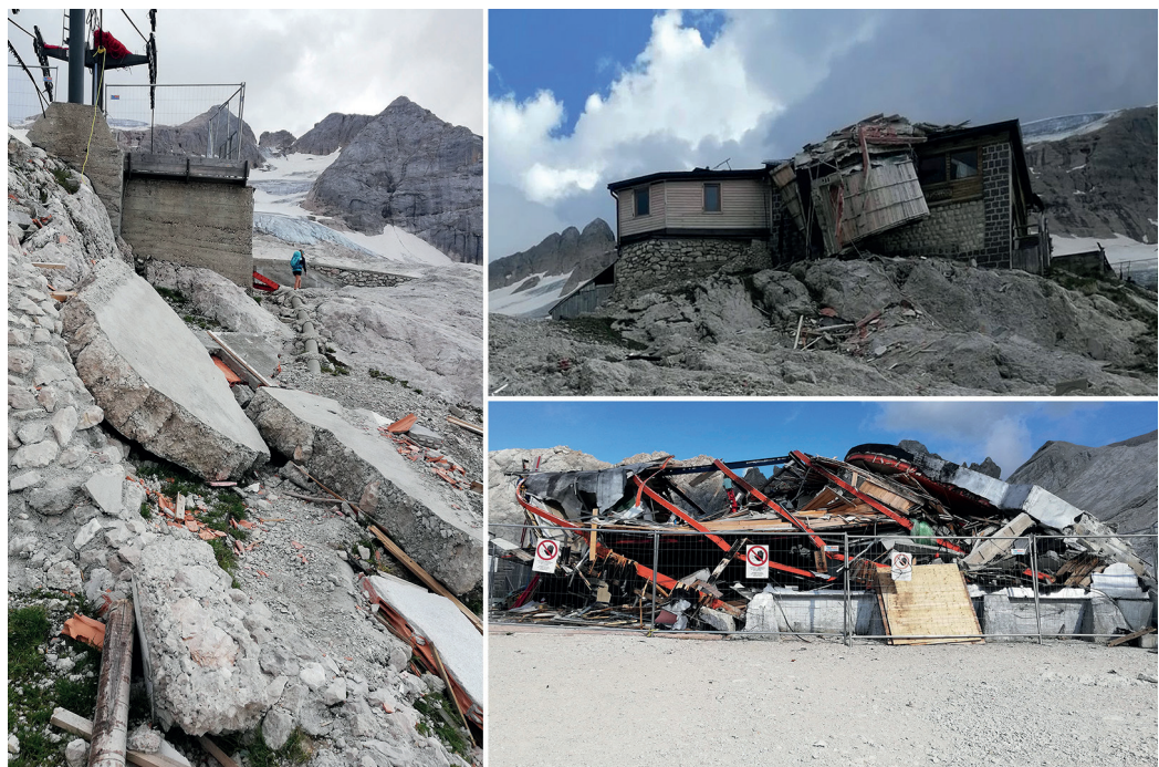
Fig. 03. The destroyed lodge (author's photo).
