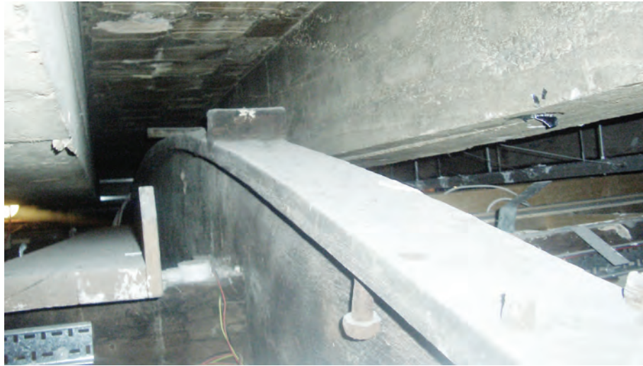
Fig. 20 The original 1848 Bramah and Robinson cast iron girders still exist today, bidden behind the plaster ceiling.
