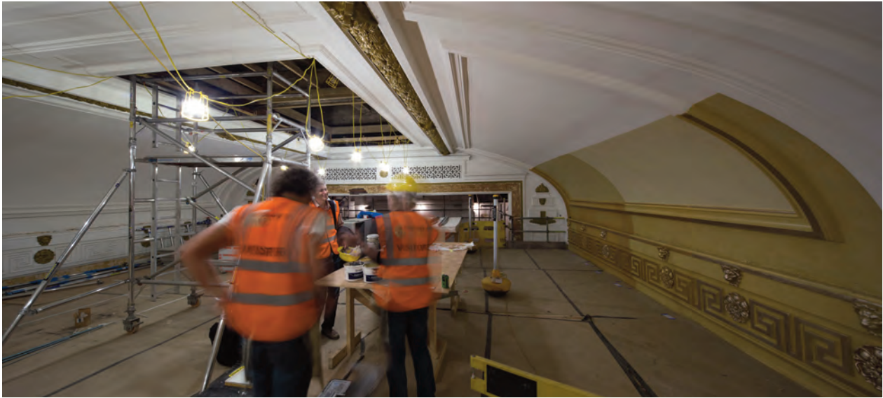
Fig. 138 The ceiling of the Regent Street Cinema during building work, October 2014.
