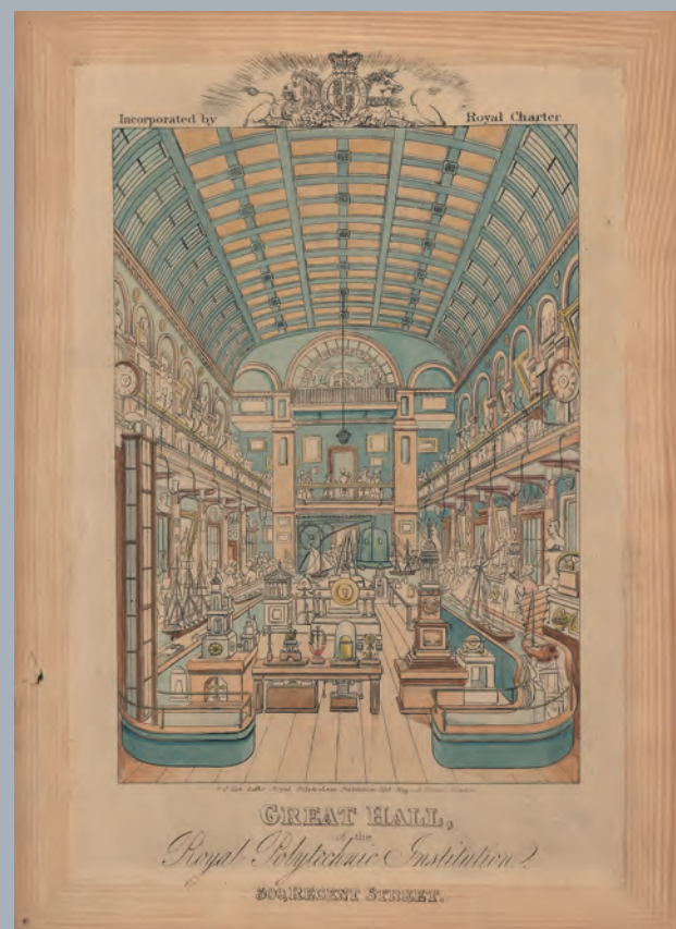
Fig. 19 The Great Exhibition Hall was 120 feet long, 40 feet wide and 40 feet high (37 x 12 x 12 m), top lit by glass panels in the curved roof.
