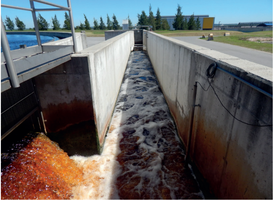
Figure 16.6 Secondary treatment at the pulp mill WWTP of study: Effluent to Uruguay River (Photo Bentancur S.).
