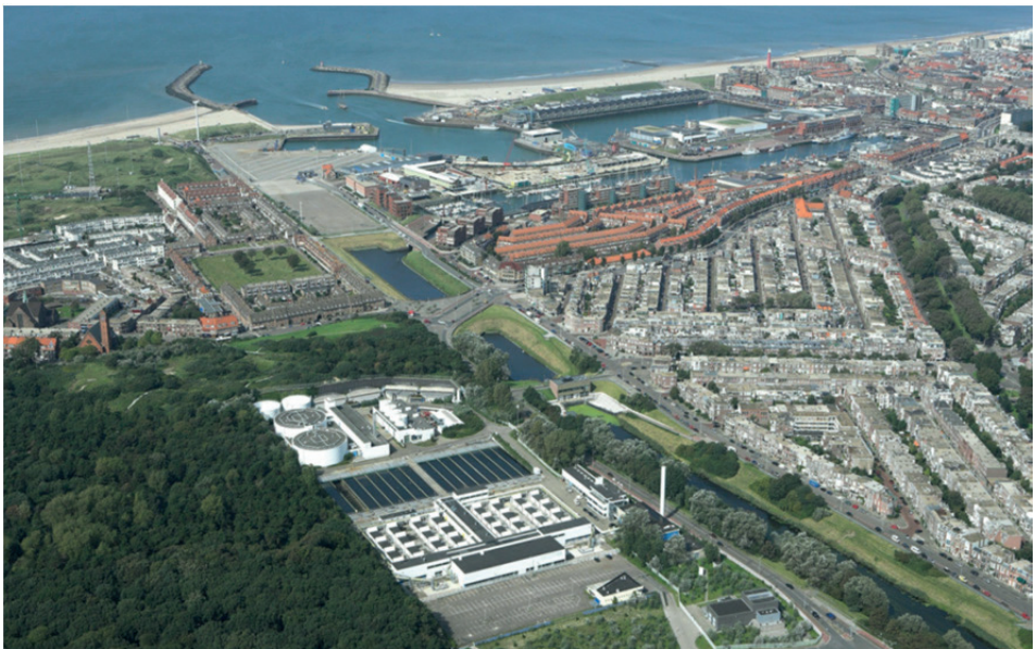
Figure 15.1 Aerial photograph of WWTP Houtrust in The Hague, The Netherlands. The Houtrust treatment plant is largely built underground. Below the parking lot are the primary setting tanks, selector, pre-denitrification, anaerobic and anoxic tanks. Eight activated sludge tanks are arranged in four lines and are covered (at the bottom of the photo). The thirty two rectangular secondary clarifier tanks are stacked in a double layer arrangement (middle section). The plant includes digestion and sludge processing (top section).
