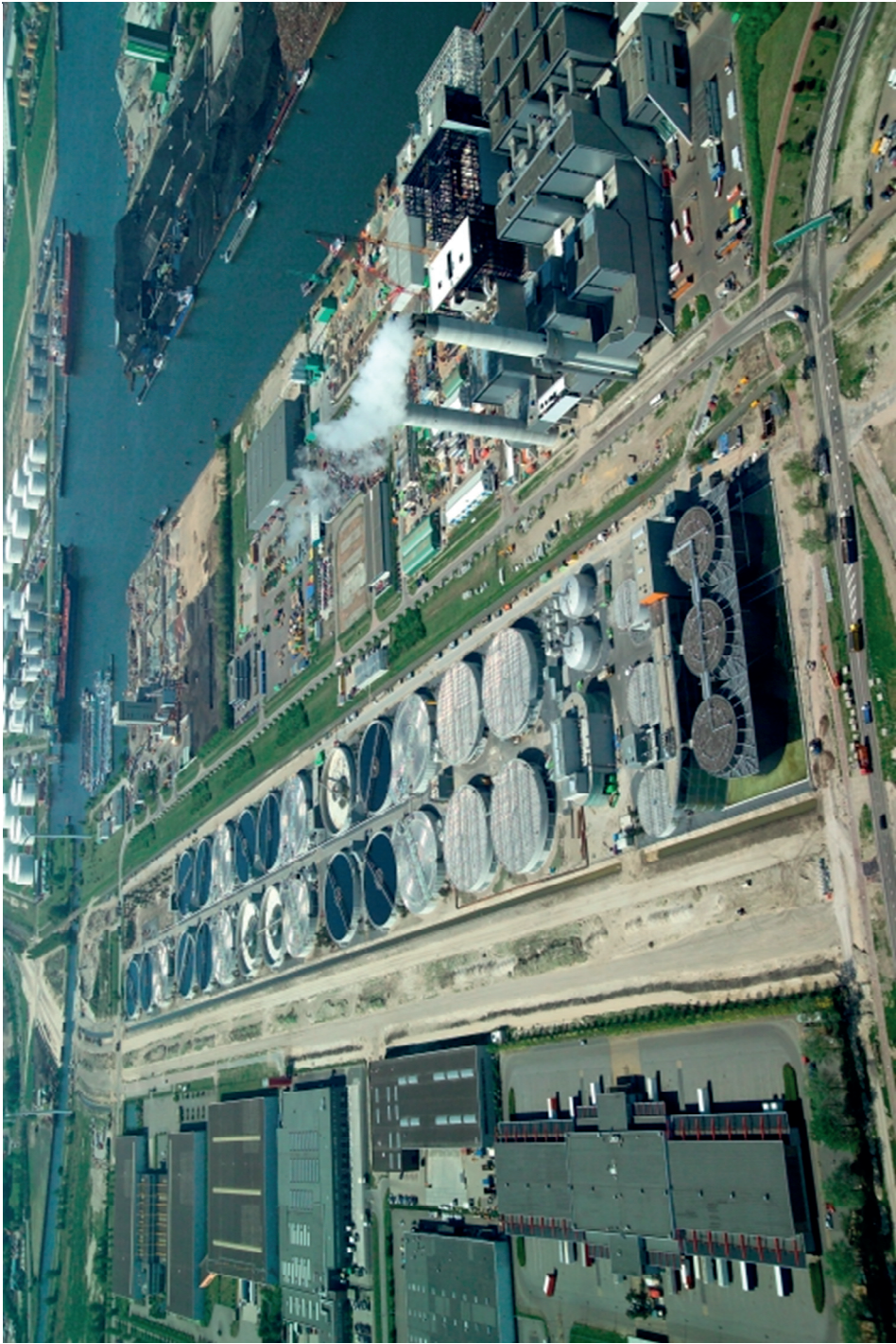
Figure 14.12 WWTP Amsterdam West (Photo: Waternet)
