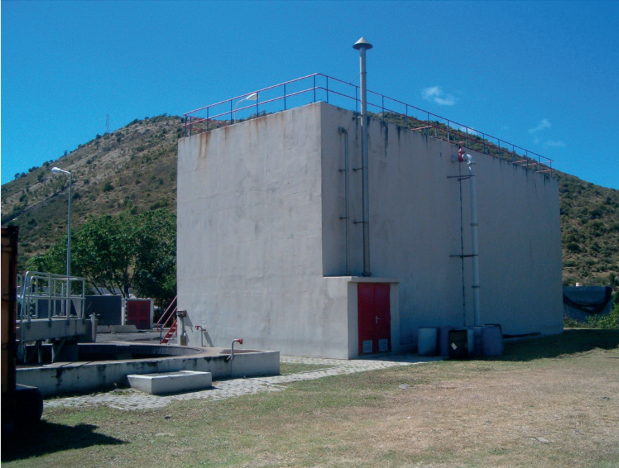
Figure 11.4 Old WWTP Illidge Rd.: biological treatment unit (Photo: Brdjanovic D.).
