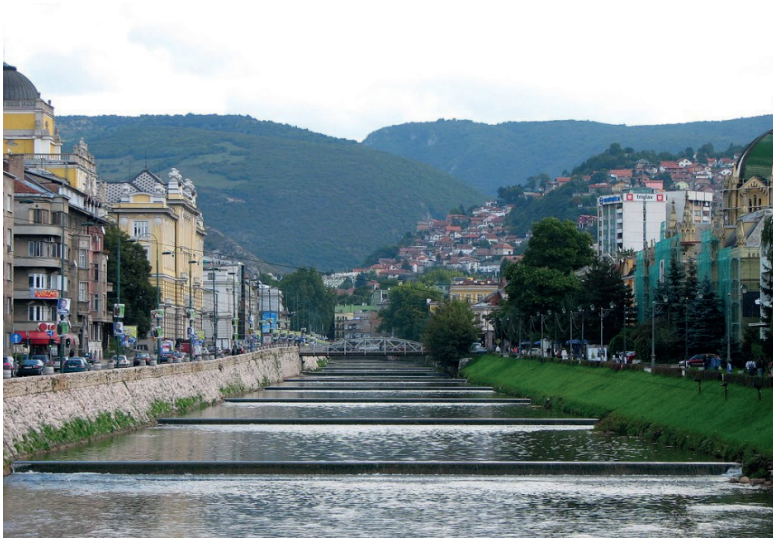
Figure 10.14 River Miljacka in Sarajevo (Photo Hodzic A.).
