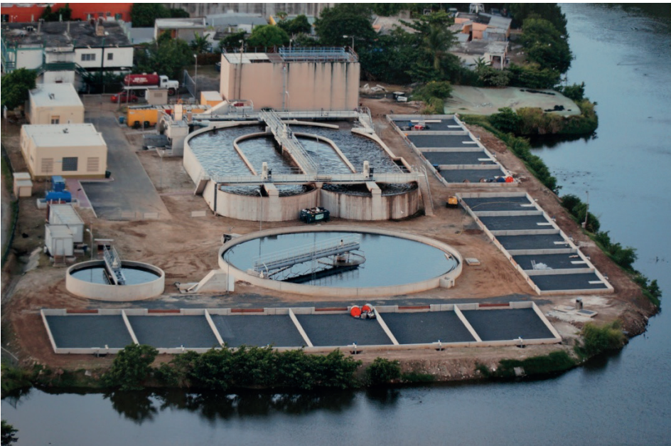
Figure 11.16 Aerial views of the old and new WWTP Illidge Rd. in operation (Photo: Buncamper C.).
