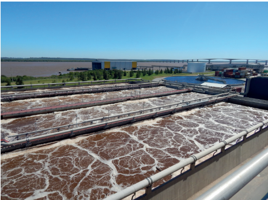
Figure 16.5 Secondary treatment at the evaluated pulp mill WWTP: Conventional aerobic activated sludge system (Photo Bentancur S.).
