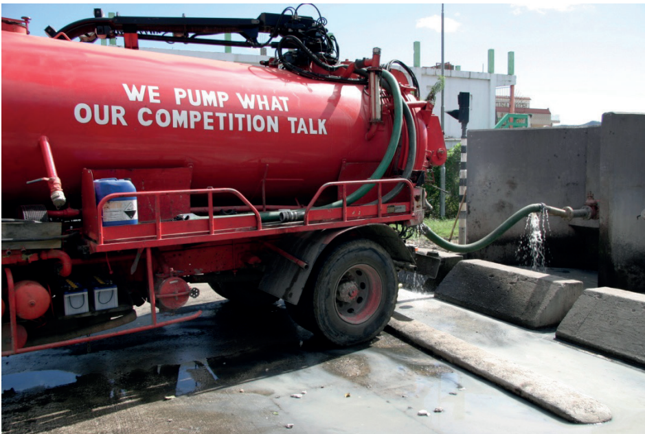
Figure 11.2 Discharge of septage to the buffer tank of WWTP Illidge Rd. (Photo: Brdjanovic D.).
