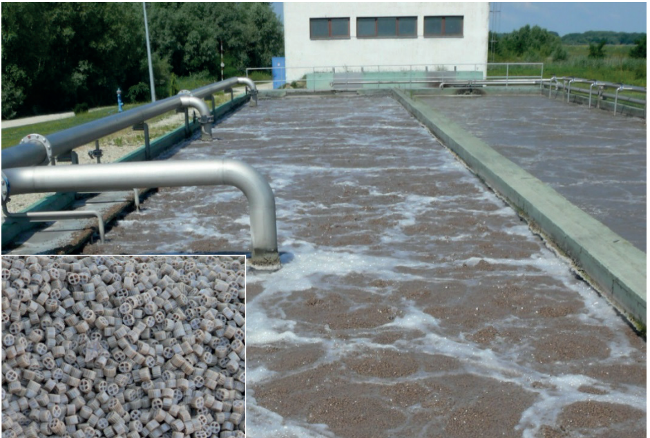
Figure 13.3 Biofilm carriers were introduced to increase efficiency of sewage treatment (photo: Brdjanovic D.).
