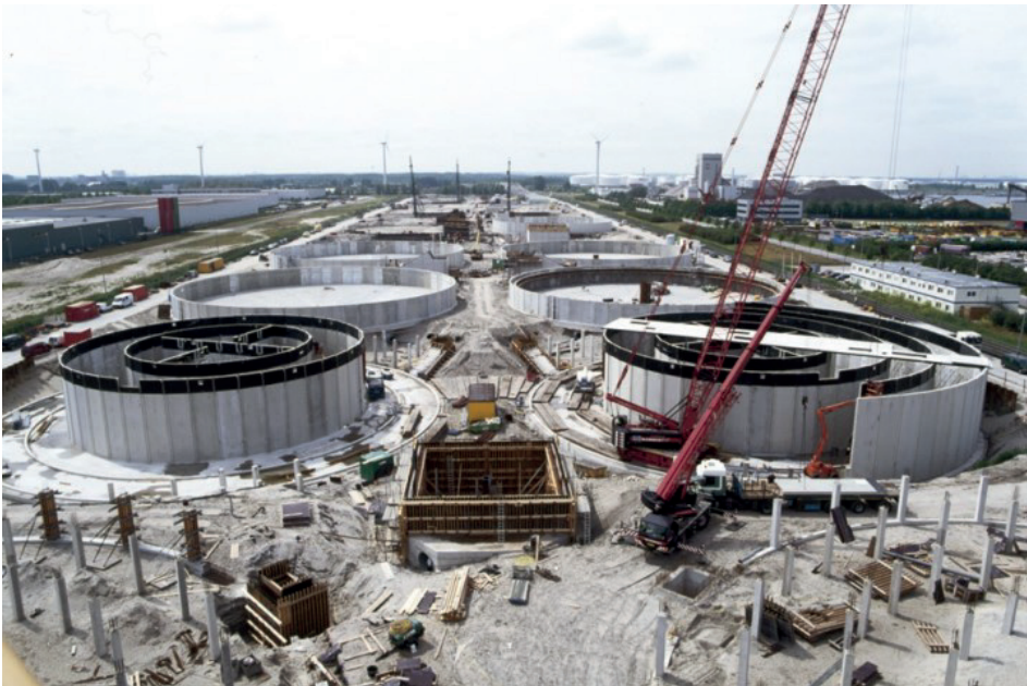
Figure 14.10 WWTP Amsterdam West during construction (Photo: Waternet)
