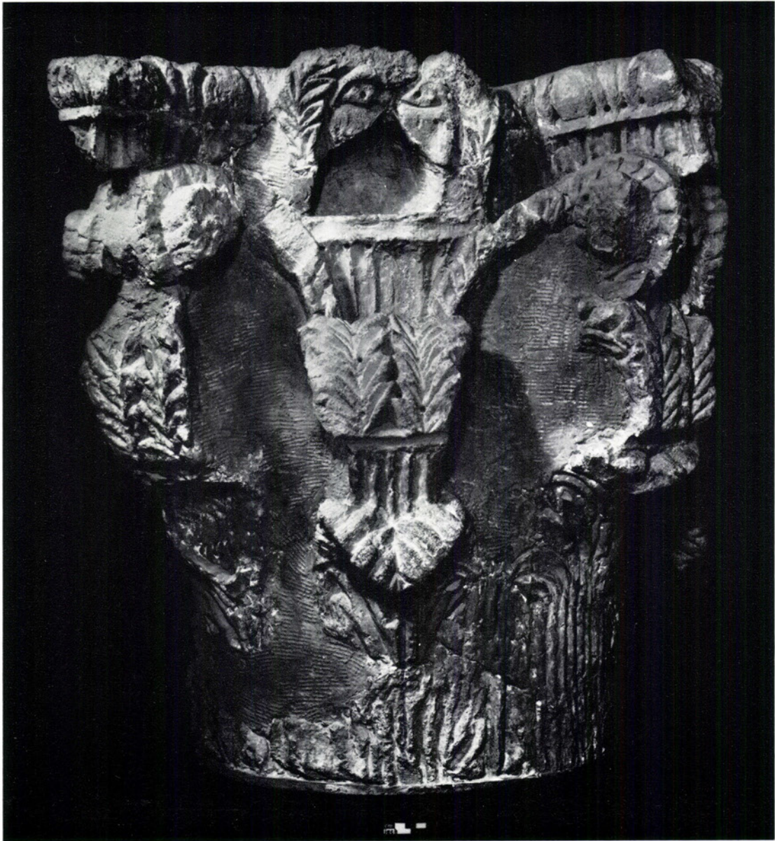
Reconstruction of a Corinthian capital using fragments of the original stonework set in a plaster backing (pp. 11-14)
