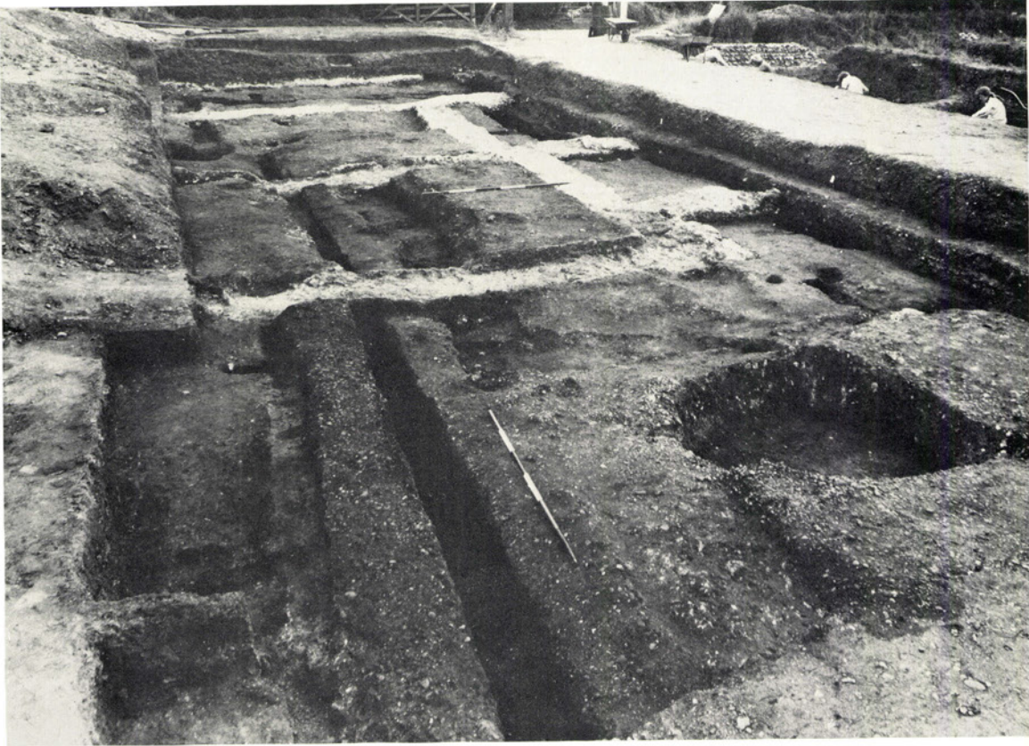
a. Chalk foundations of Building XIV 7, looking N.E., with II D plank-lined drain (centre) and Wall 55/56 (left foreground) (pp. 9, 76)
