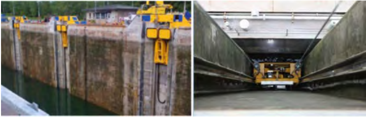
Fig. 11. The vacuum-type automatic floating mooring system
