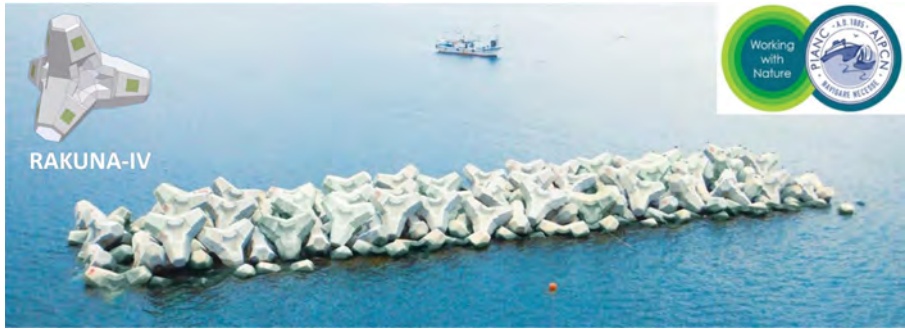
Photo 1. EAC Demonstration experiment in the construction of the 6 th breakwater at the port of Wajima (PIANC Working with Nature Certificate of Recognition)
