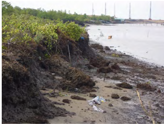
Fig. 3. Condition of river bank
