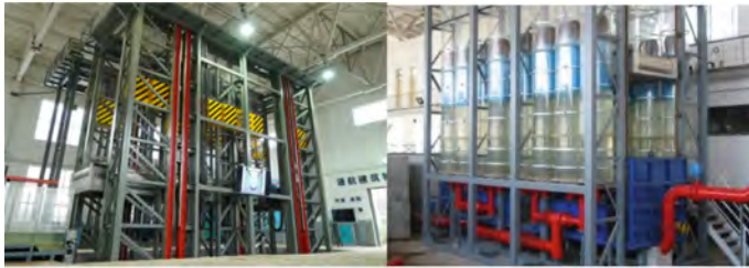
a) Rack and pinion ship lift (3000t)
