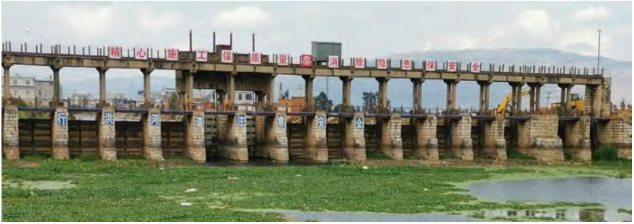
Fig. 4. Xinba sluice on the Laopanjiang River
