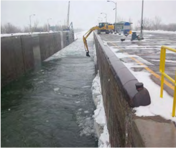
Fig. 3. Ice removal with long arm excavator
