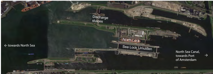
Fig. 1. IJmuiden lock complex, with the names of the most important elements indicated (Google Earth).
