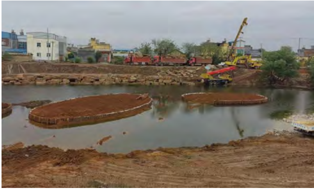
Fig. 8. River shoals under construction
