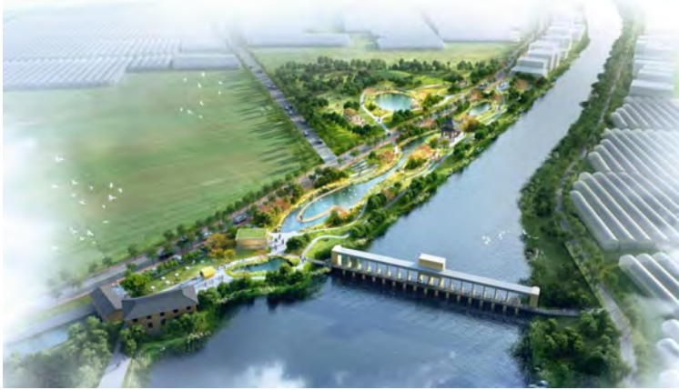
Fig. 9. Aerial view of water moistening everything node
