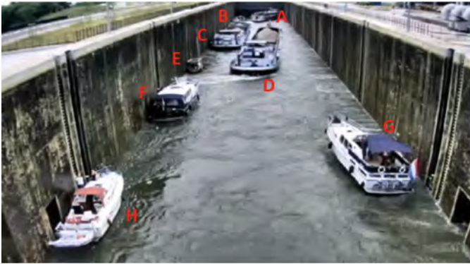
Fig. 2. Asymmetrical filling at the lock of Lanaye
