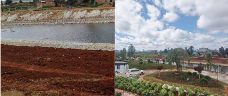
Fig. 2. Aerial view of new embankment
