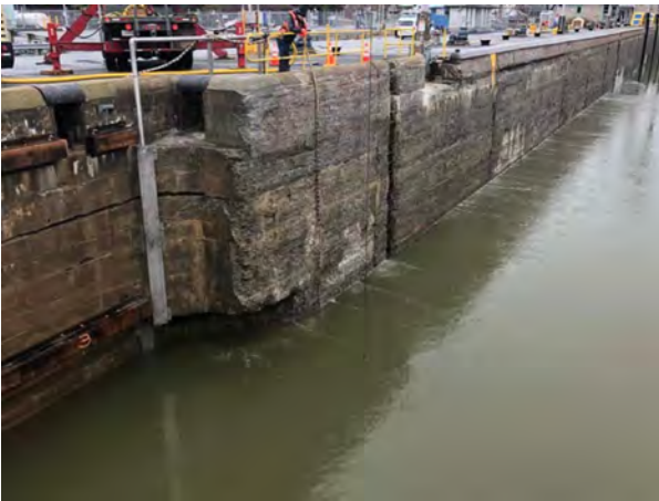
Fig. 15. Pilot longitudinal bubbler system in operation at St. Lambert Lock. Note bubble plumes visible along the lock wall.
