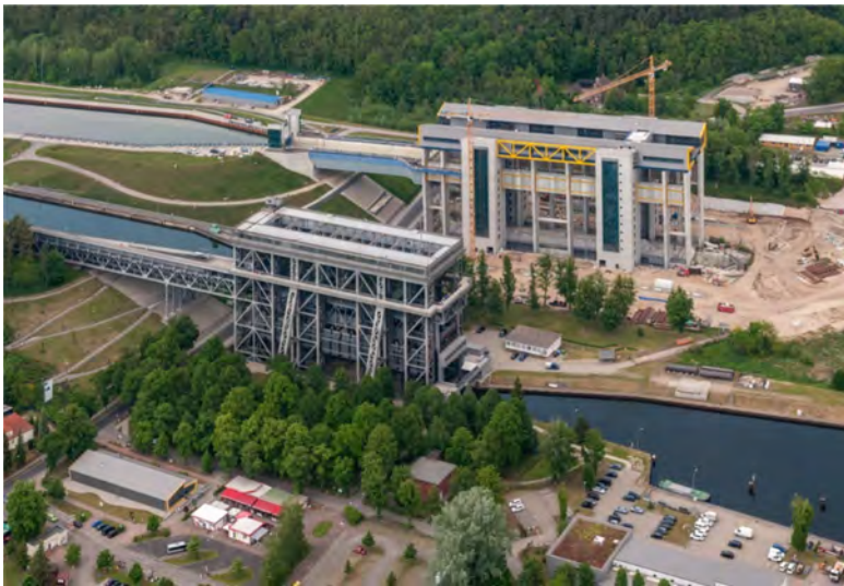
Fig. 15. New Niederfinow Ship Lift and Old Niederfinow Shiplift
