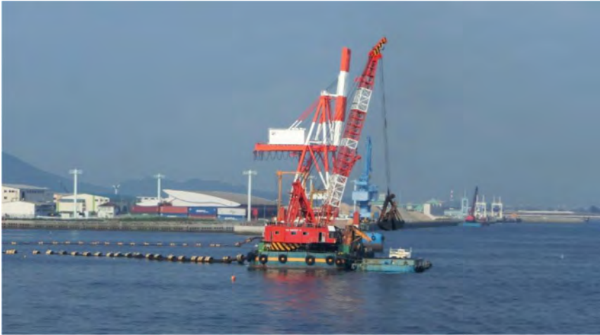
Fig. 7. Work status of dredging
