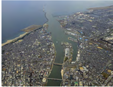
Fig. 2. Aerial photo of the port area.
