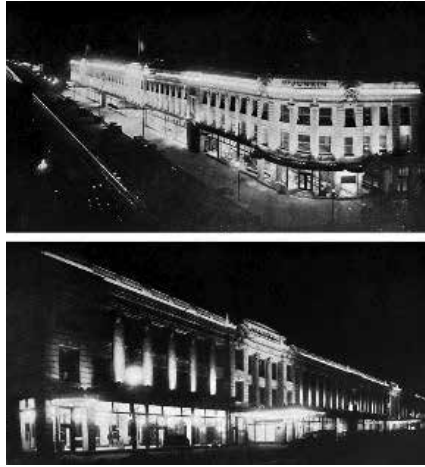
Figure 12. Night views of the McJunkin Building, Chicago. Flashers and contact board produce different effects: white light on pilasters and colored lights on the bays between pilasters in the top image; “clear flux” on pilasters only and a cornice band of golden light combine to give “the effect of a Greek Colonnade”
