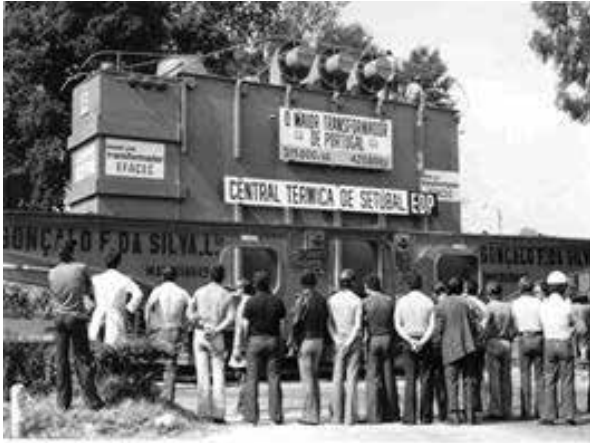
Fig. 2. Delivery of an EFACEC transformer, considered “the largest transformer made in Portugal” and destined for the Central Térmica de Setúbal
