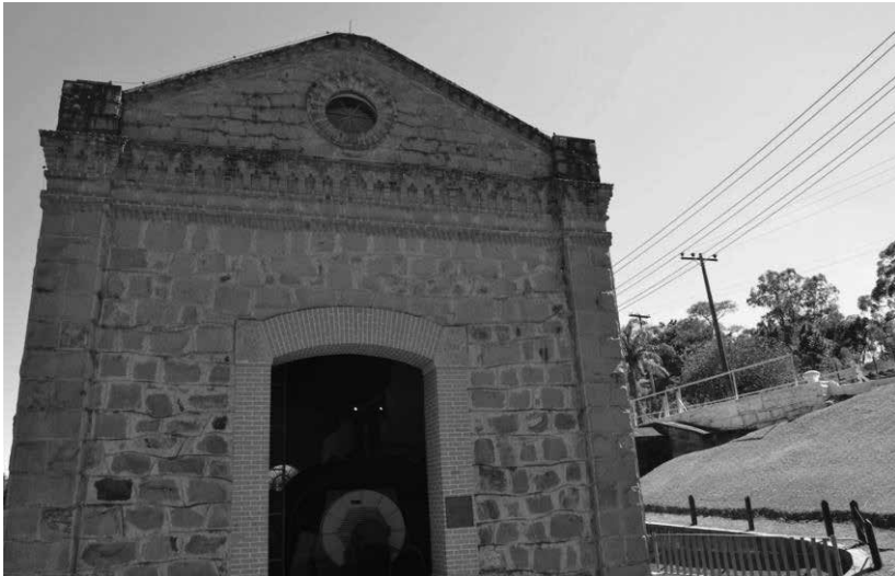
Figure 2. Salto Grande power station (built in 1906)
