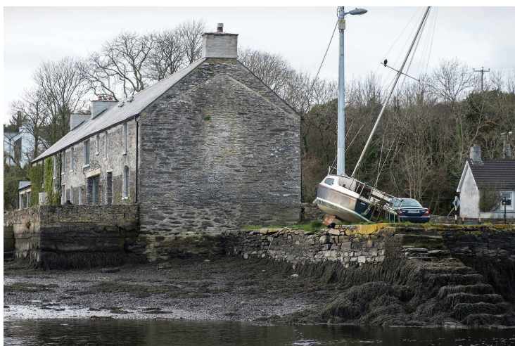
Figure 7.7 The original pitch line of the roof of the warehouse and the outline of the crane door can be discerned. Photograph by Kevin O’Farrell 2021.
