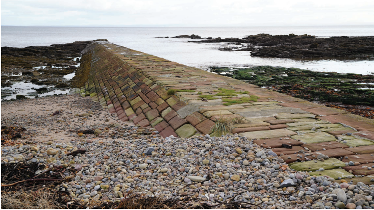
Figure 3.3 Rockfield pier: protective slope. Photograph by Hilary Wyatt 2022.
