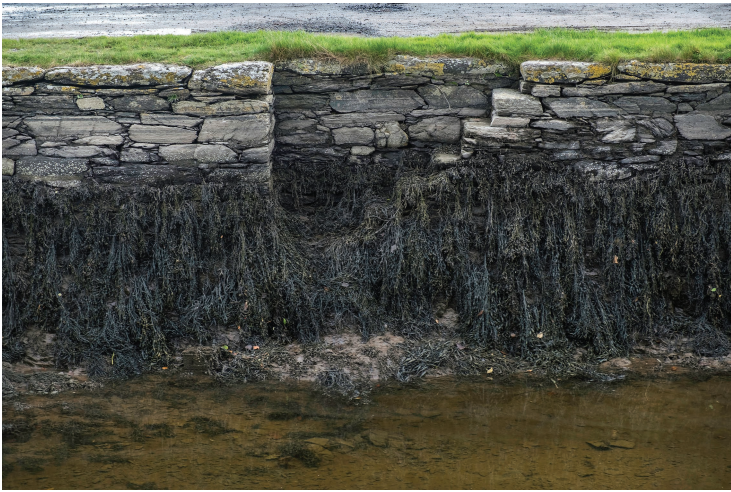
Figure 7.6 A detail of the Quay wall showing pinnings and traces of lime mortar. Photograph by Kevin O'Farrell 2021.
