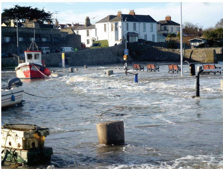
Figure 1.1 Bullock Harbour (Ireland) main pier and quay edge overtopped at extraordinary high tide. Photograph by Eamon McElroy, Chief Engineer, Dublin Port, 2014. Reproduced courtesy of the Dublin Port Archive.
