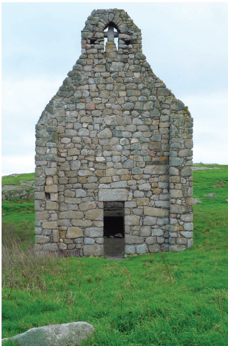
Figure 5.3 Record photograph of the west face of St Begnet's Church, Dalkey Island, 9th century. This flat on image could be scaled to produce a rectified elevation. Photograph by Bill Hastings.
