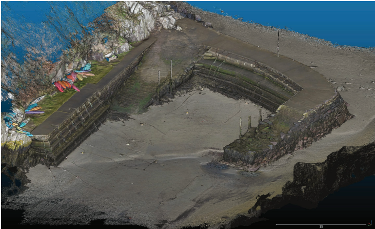
Figure 4.4 NPRN 34342, Porthclais harbour. 3D model derived from a combined laser scan and drone-based photogrammetry survey undertaken by the RCAHMW on 20 February 2023 (© Crown copyright: RCAHMW).
