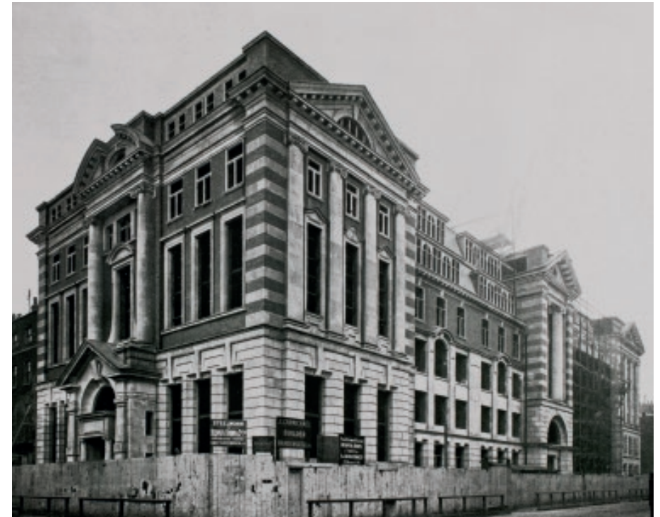
Fig. 5.3 The new Medical School almost ready for opening in 1907.
