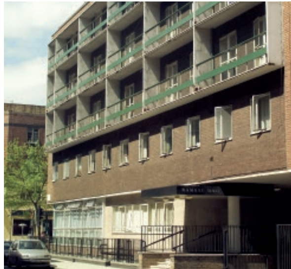
Fig. 7.13 Ramsay Hall, a large hall of residence only five minutes walk from the main UCL campus, was opened in three stages between 1964 and 1987.
