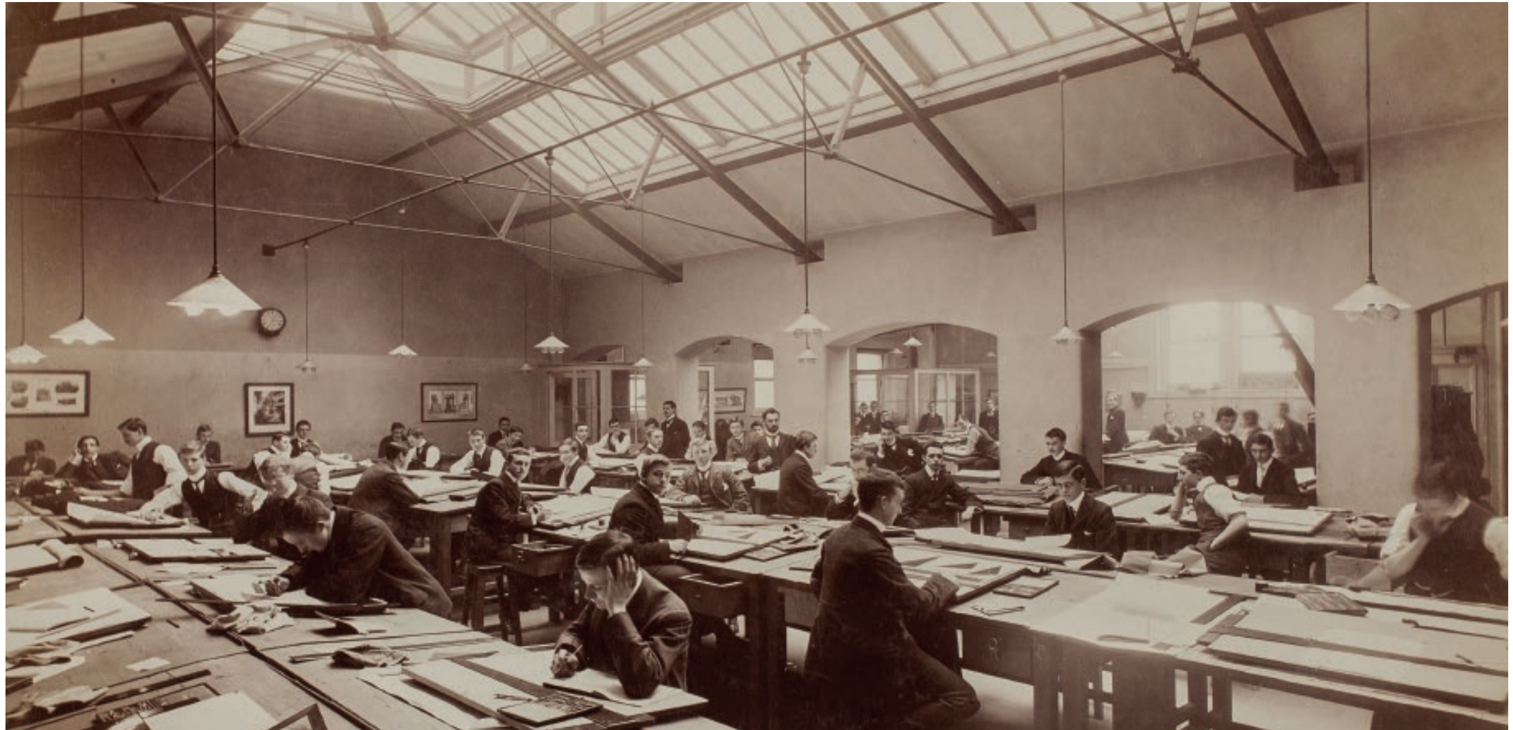
Fig. 4.15 The Drawing Office on the top floor of the Engineering Building long desired by Kennedy, soon after its eventual construction in 1893.
