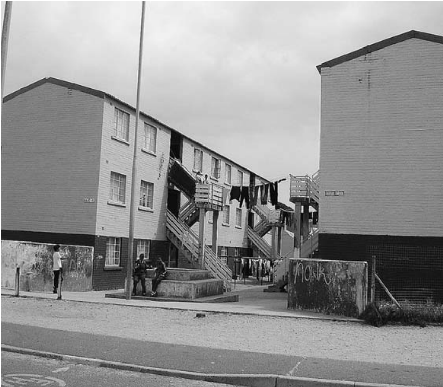
Housing in a coloured township on the Cape Flats, 2006. Constructed after the forced removals under the Group Areas Act in Cape Town in the 1960s and 70s, such sub-standard housing is found in all coloured townships on the Cape Flats.
