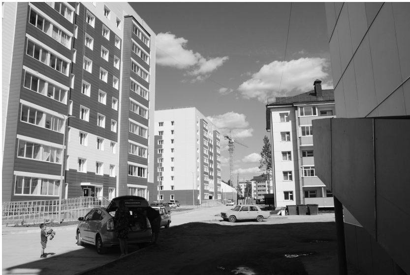
Figure 7.1 Young family moving in one of the new apartments in Neryungri, Churapchinskaia Street.
