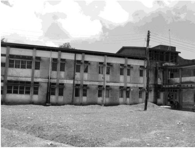
Figure 3: Care and Treatment Center of Bombo Regional Hospital (Personal photo, 2008).
