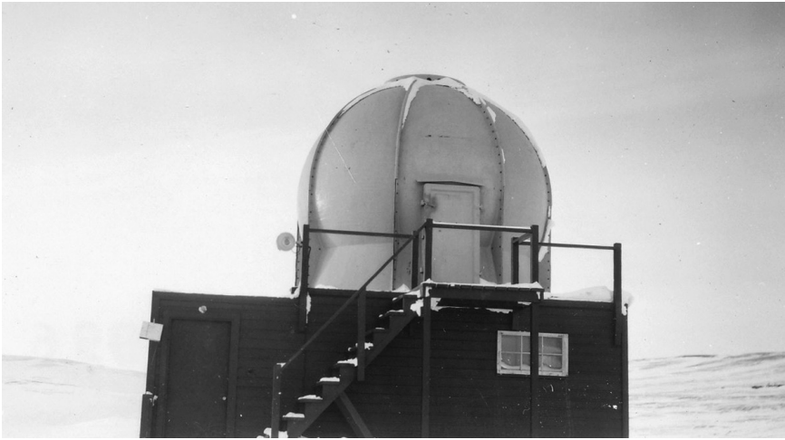
FIGURE 6-4. The rawinsonde building at Mould Bay in the mid-1950s. Note the light on the left side of the porch. Jim Jung Collection.
