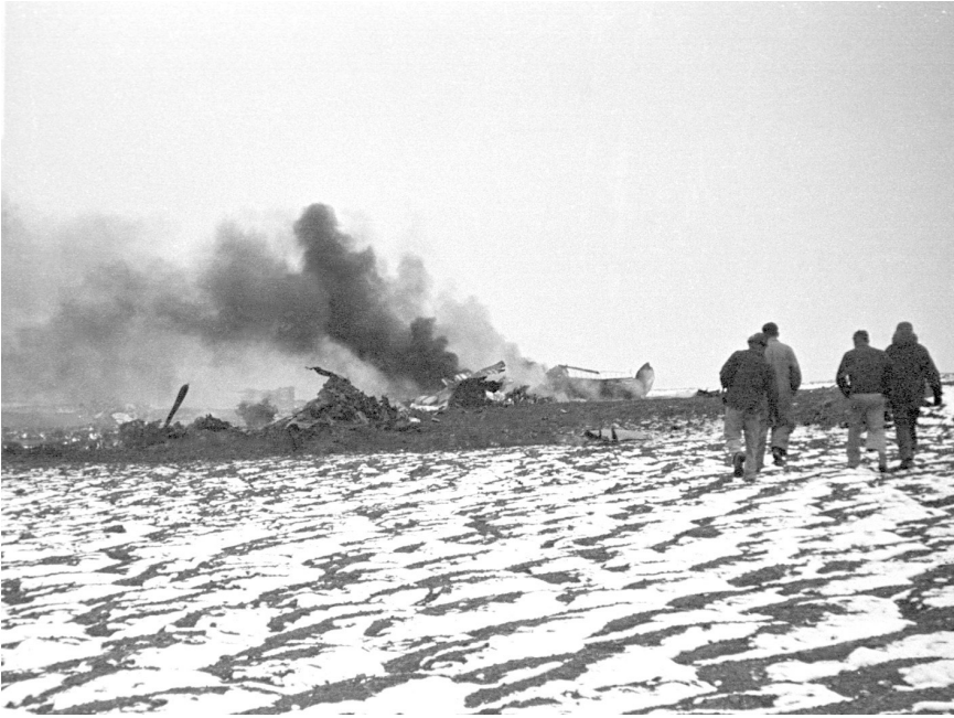
FIGURE 4-11. Station personnel approach the crash site, 31 July 1950. Pete Johnson Collection.
