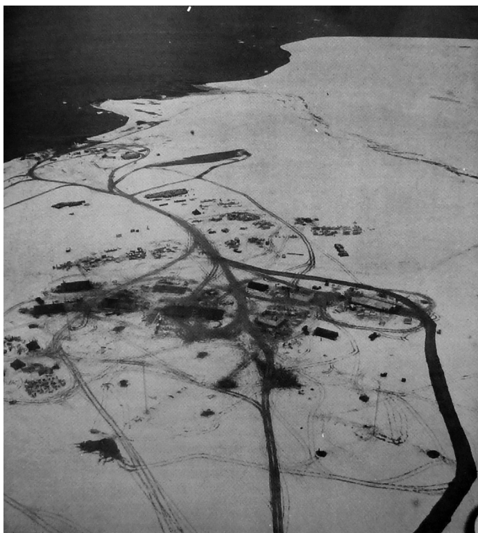
FIGURE 3-10. Resolute Bay under construction following the season's first snowfall, 10 September 1947. United States Navy Department.
