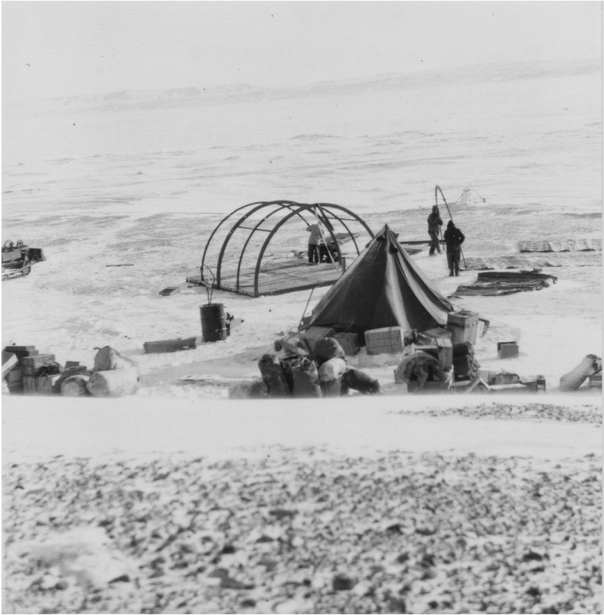
FIGURE 3-3. Personnel erecting the Jamesway hut on their first day at Eureka, 8 April 1947. John Trinko family collection. Published with permission of the Trinko family.
