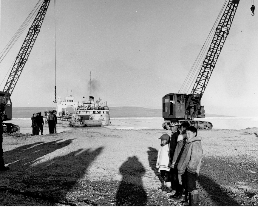
FIGURE 7-5. Inuit were not passive observers during the sealift. Many men worked as shore hands, but the research for this book did not uncover any photographs of their contributions. LAC R184, RG12, Acc. 1982-241 NPC, Box 192, 1940, 3857, C 0346--C 0349 3858 OS 0059.
