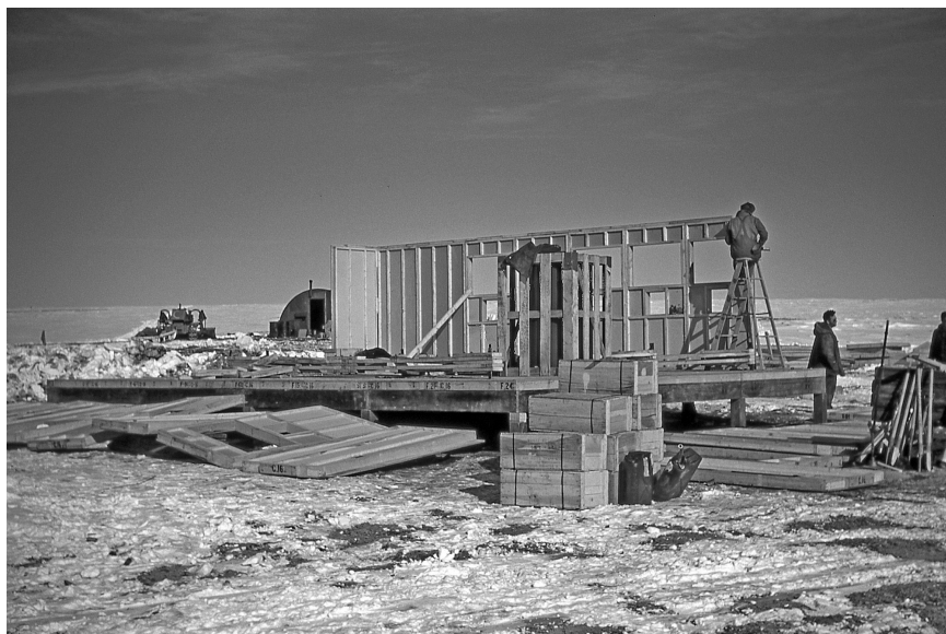
FIGURE 4-10. Erecting the walls of Alert's operations building, 13 May 1950. Peter Johnson Collection.
