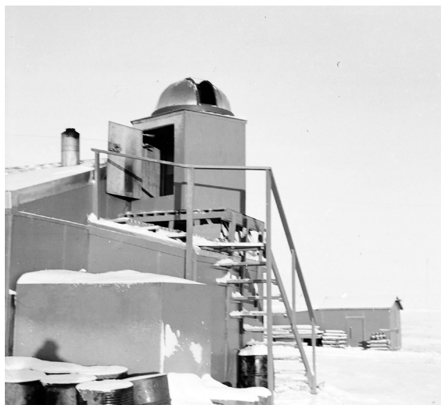
FIGURE 6-7. The PIBAL dome at Isachsen in 1953. Despite the dome, the unheated space meant that PIBALs remained among the least-liked observations that station personnel had to conduct. Bill Nemeth Collection.
