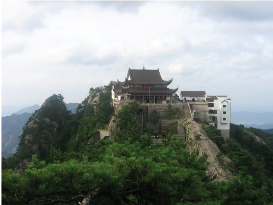
Fig. 37. Treasure Hall of the Great Hero ( Daxiong baodian 大雄宝殿) at Mount Juhua. 231
