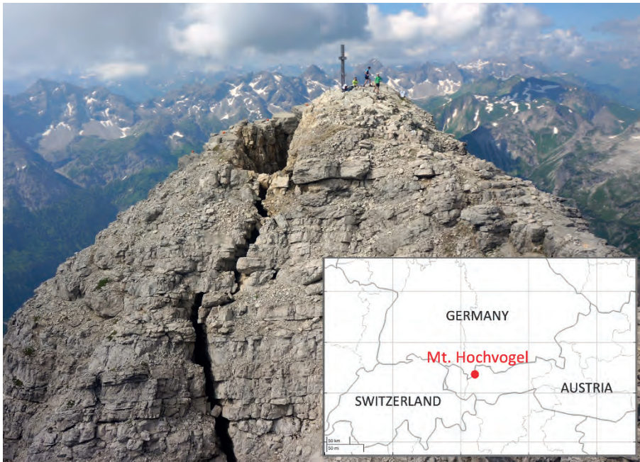
Figure 1: Mt. Hochvogel (2592 m a.s.l.) is one study site within the research project AlpSenseRely where new geo-monitoring strategies are developed and tested.
