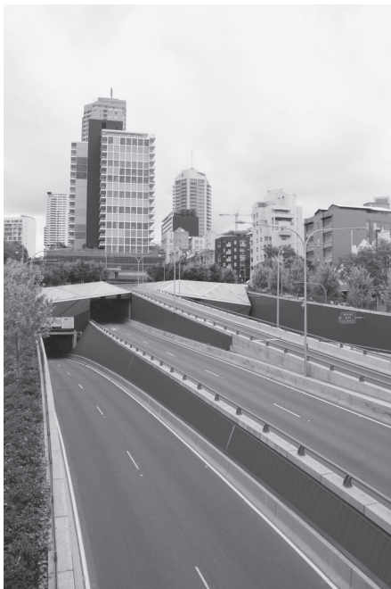
Figure 10.1 Photograph of the Cross City Tunnel (Judd 2008) (with permission from Trafford Judd)
