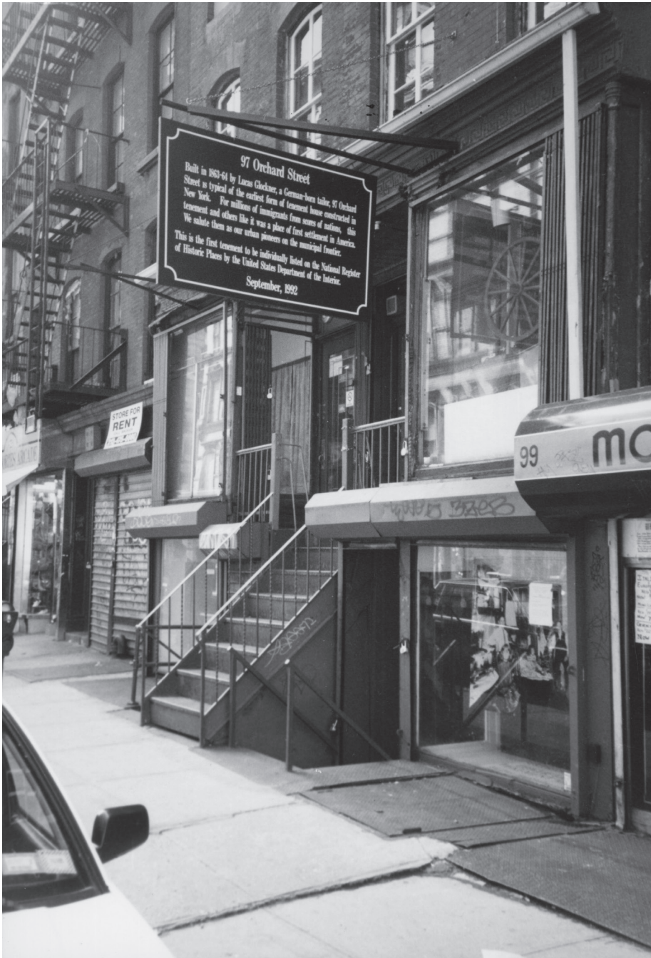
Facade of 97 Orchard Street, ca. 1994. Collection of the Lower East Side Tenement Museum.
