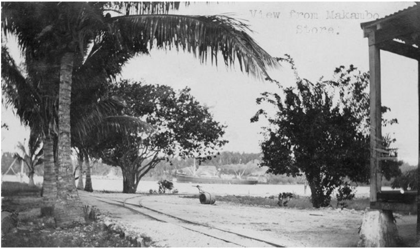
Plate 2.10 BP's Makambo Island, showing the rail system that transported supplies to and from the wharf. Tulagi is in the background Source: NBAC, N115-520.
