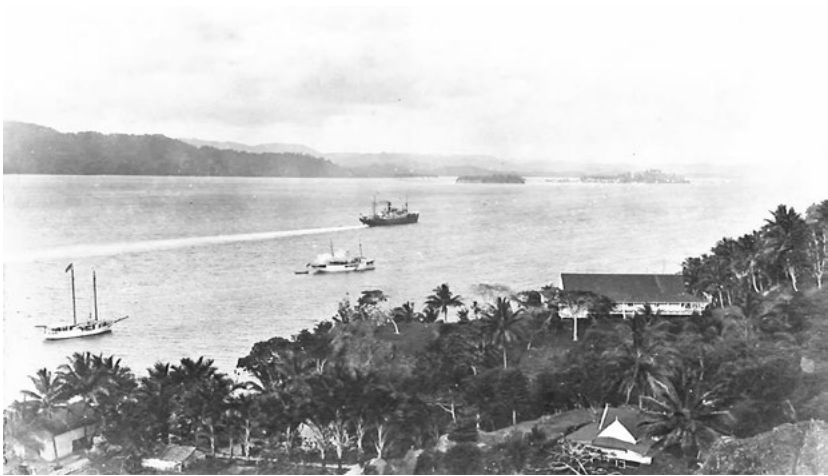
Plate 2.13 BP's SS Mataram sailing from Tulagi Harbour for Sydney
