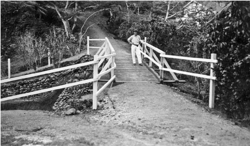
Plate 3.4 The bridge over the cutting enabled easy contact between all residents on the ridge
