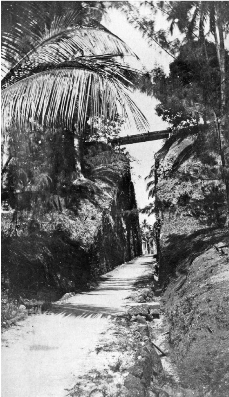
Plate 3.3 The completed cutting, showing the bridge over the top Source: UQFL, Wilson Papers and Photographs.
