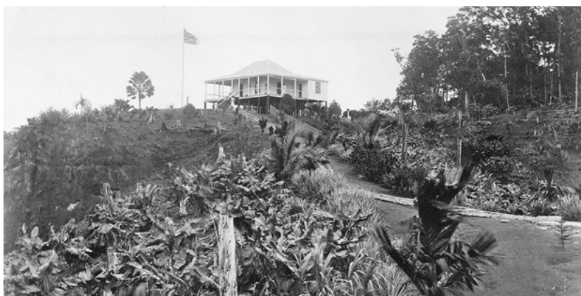
Plate 2.2 The first residency, built in 1898 on Tulagi's central ridge
