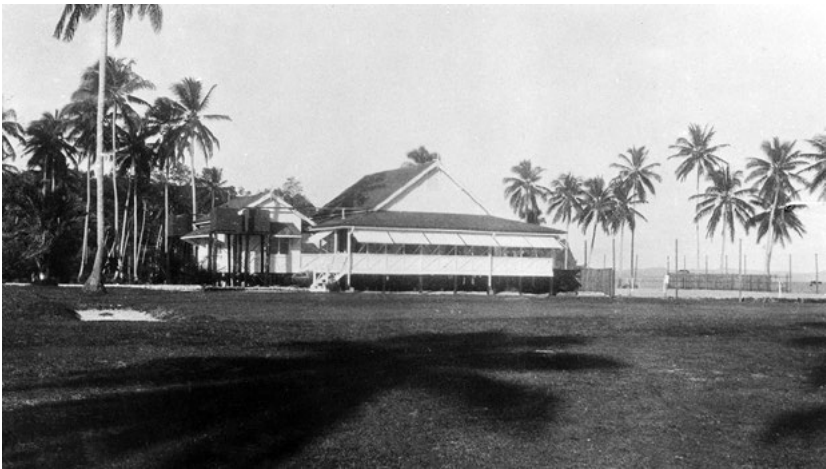
Plate 4.4 The Tulagi Club, 1930s. Shutters and sides have been added to enclose the verandah
