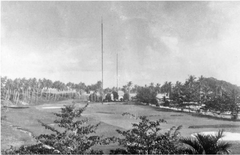
Plate 4.9 The two wireless station masts and the golf course, 1930s
