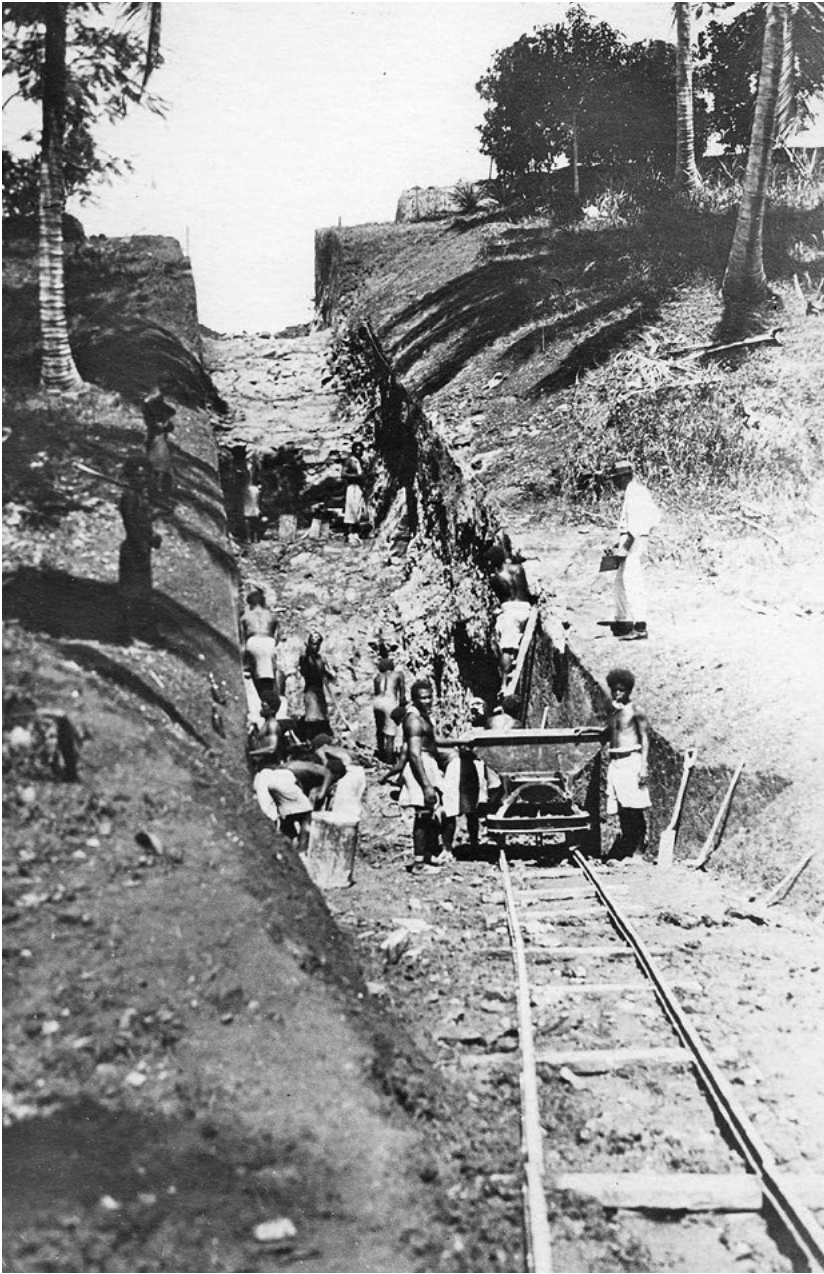
Plate 3.2 The cutting through the central ridge was constructed in 1918 using prisoners and indentured labourers
