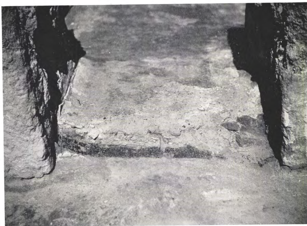
b. Room 9, the doorway, showing wooden sill-edge and the packing of the raised threshold p. 120
