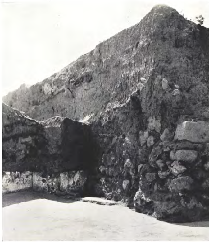
a. The foundations of the NE. corner cut down into room 2 of the Level VII palace
