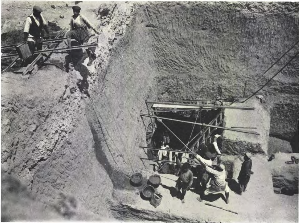
a. Excavations of 1947; digging below water-level p. 36
