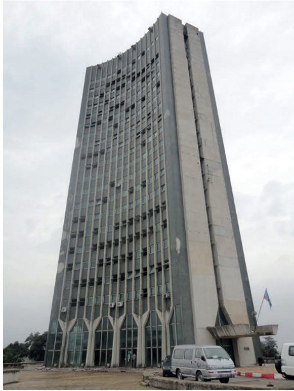
Fig. 27. CNRT Tower, Kinshasa, 2014 (Photograph © Ruth Sacks.)
